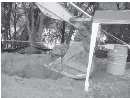
Test pit during Phase I drum removal.
