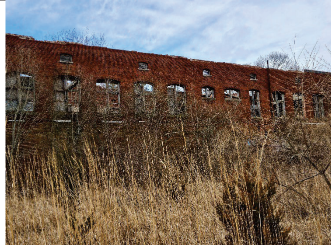
Back of Building – Note roof missing
