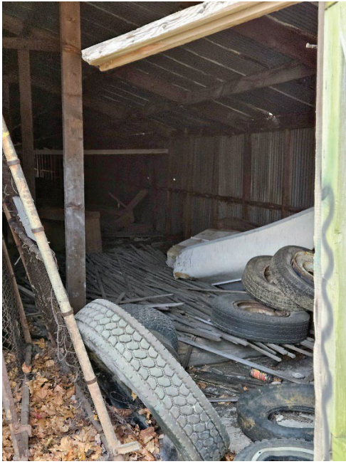
Inside Metal Shed
