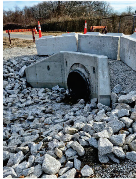
New Culvert under Bike Path
