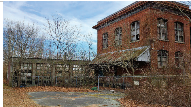
Left side of Building
