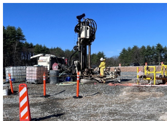
Drill rig and injection mixing station set-up for microscale zero-valent iron injections
