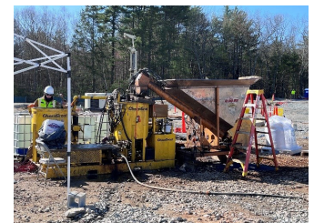
Drill rig and injection mixing station set-up for microscale zero-valent iron injections
