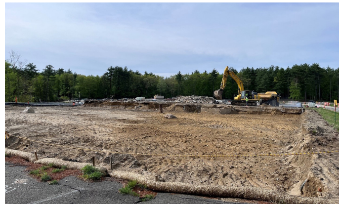
Building D excavation area
