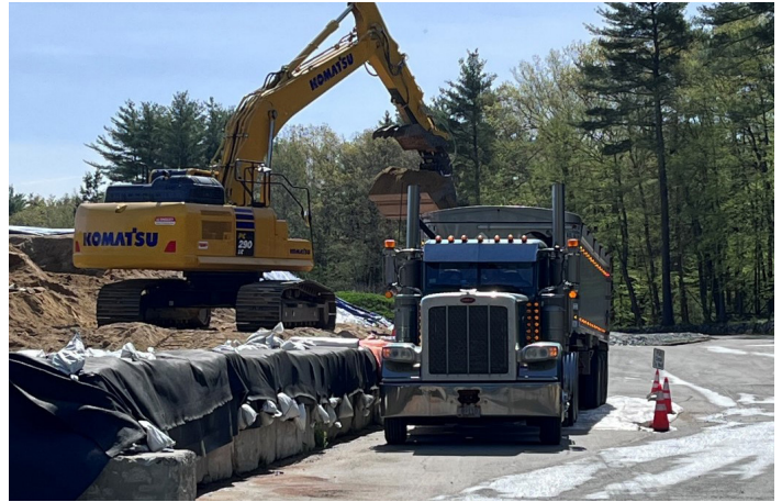
Photo 8: Soil is trucked from Concord, Mass. to Worcester, Mass. where it is transferred to a rail car for final transportation and disposal in Michigan at an EPA approved and licensed disposal facility.
