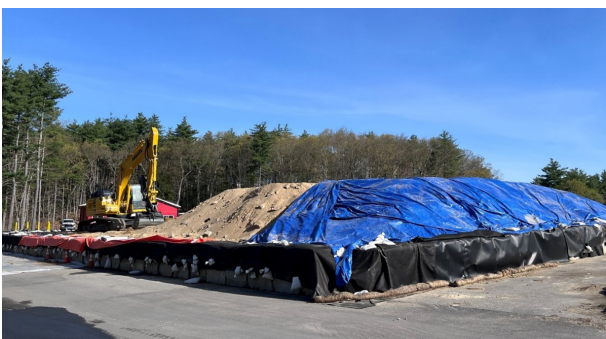
Photo 5: The Waste processing area (WPA) is where soils are temporarily stockpiled before being loaded into trailers for off-site disposal.
