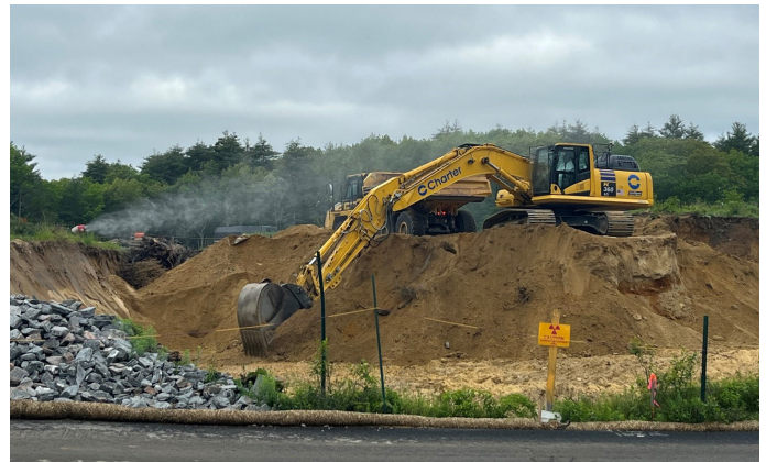
Excavation of the former Courtyard area
