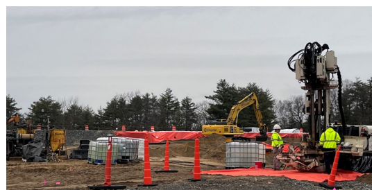
Drill rig set-up for microscale zero-valent iron injections
