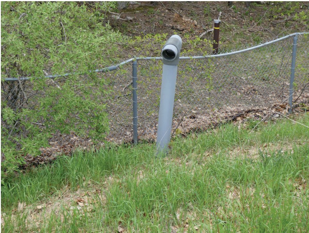
Gas vent and monitoring well in southeast corner of landfill
