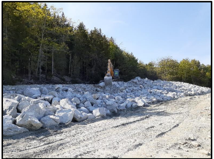
Photo 4 (group). Views of Western Ore Pad slope during 36" rock placement.
