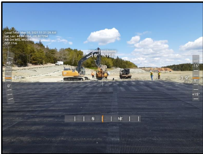
Photo 5 (group). Views of Southwest corner geo-grid and fines placement as surface stabilization.
