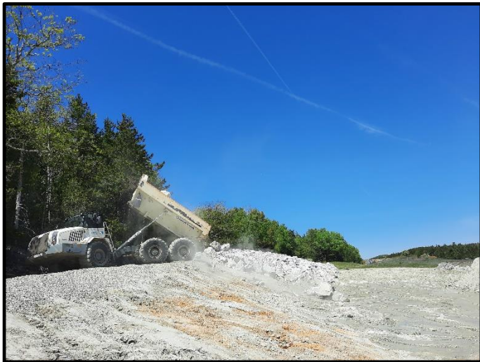
Photo 4 (group). Views of Western Ore Pad slope during 36" rock placement.
