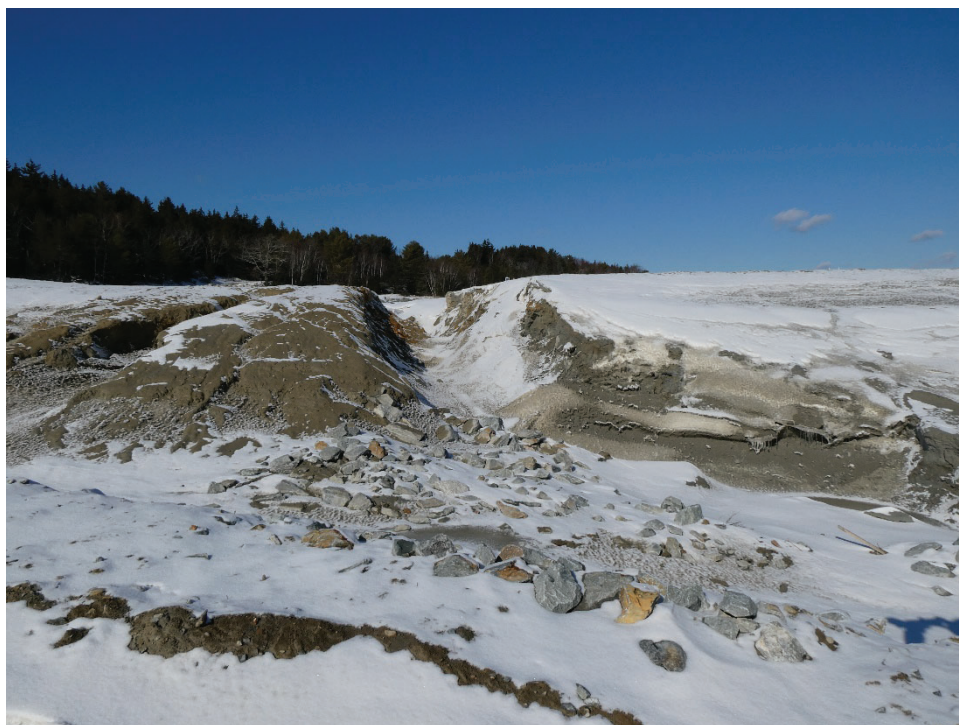
Erosion on Tailings Impoundment
