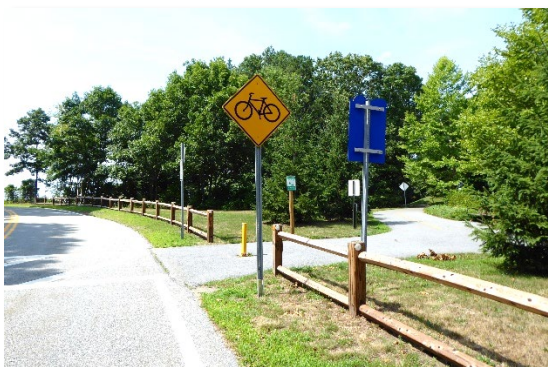
Figure 21. Quonset Davisville Bike Path.
