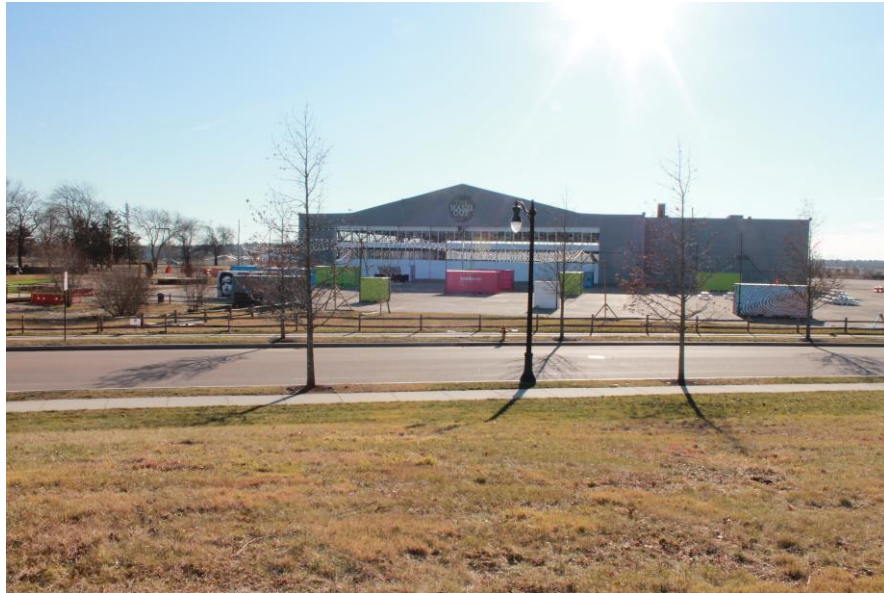
Date: 12/5/2018 Picture No. 5 Location: Building 82 Comment: Hangar 2 and northern portion of site from Memorial Grove Ave., looking south
