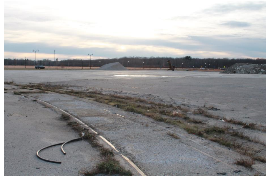
Date: 12/5/2018 Picture No. 2 Location: Hangar 1 Comment: Western portion of AOC Hangar 1
