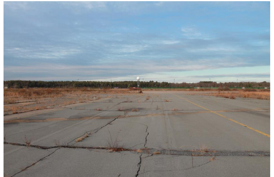
Date: 12/5/2018 Picture No. 4 Location: FFTA Comment: Looking north from FFTA up Taxiway C
