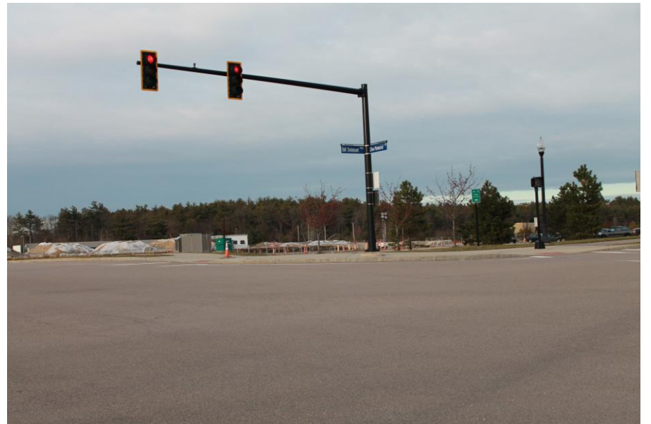
Date: 12/5/2018 Picture No. 12 Location: Hangar 1 Comment: NE portion of Hangar 1 area and intersections of Shea Memorial Dr. and Bill Delahunt Parkway
