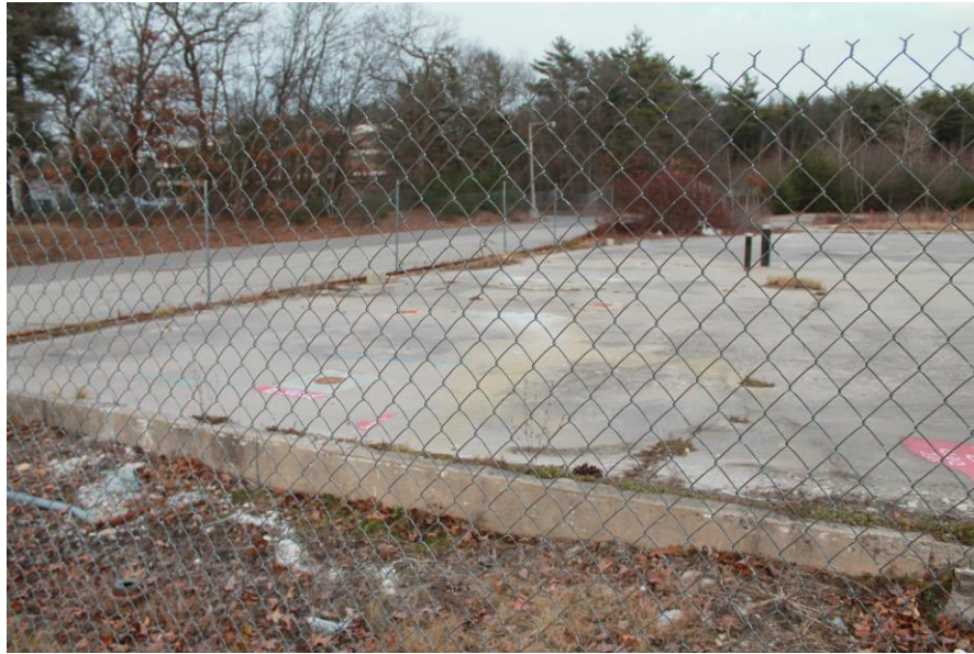
Date: 12/5/2018 Picture No. 21 Location: Building 81 Comment: View of northern portion of Building 81 area, looking northeast
