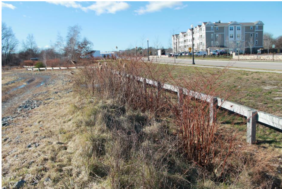
Date: 12/4/2018 Picture No. 31 Location: WGL
