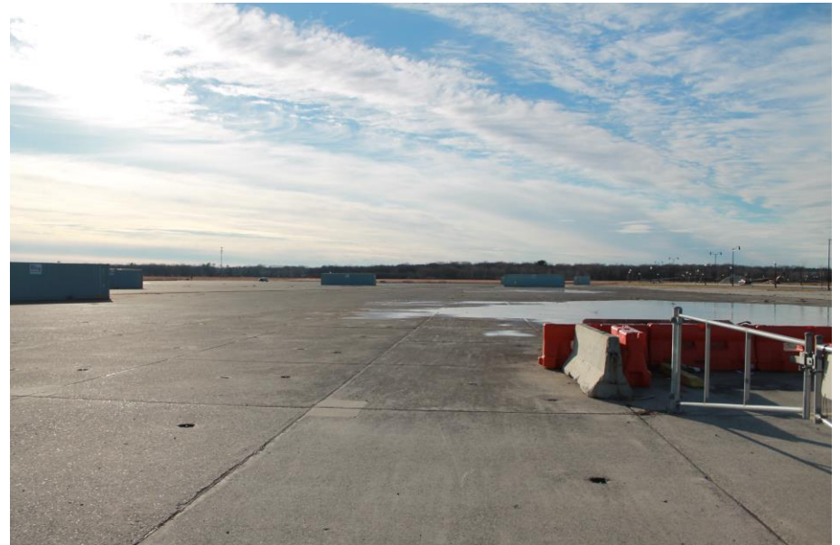
Date: 12/5/2018 Picture No. 20 Location: Hangar 1 Comment: View of southern portion of AOC Hangar 1, south of Patriot Parkway, looking west
