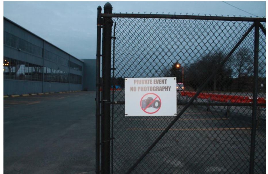
Date: 12/5/2018 Picture No. 4 Location: Building 82 Comment: Fence surrounds Building 82 site area but gates are open, unrestricted
