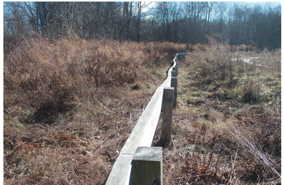
Date: 12/4/2018 Picture No. 32 Location: WGL
