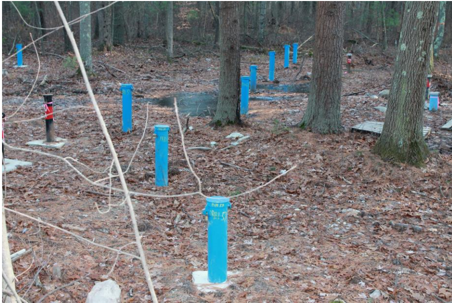
Date: 12/6/2018 Picture No. 17 Location: SRA Comment: View of PRB1-57
