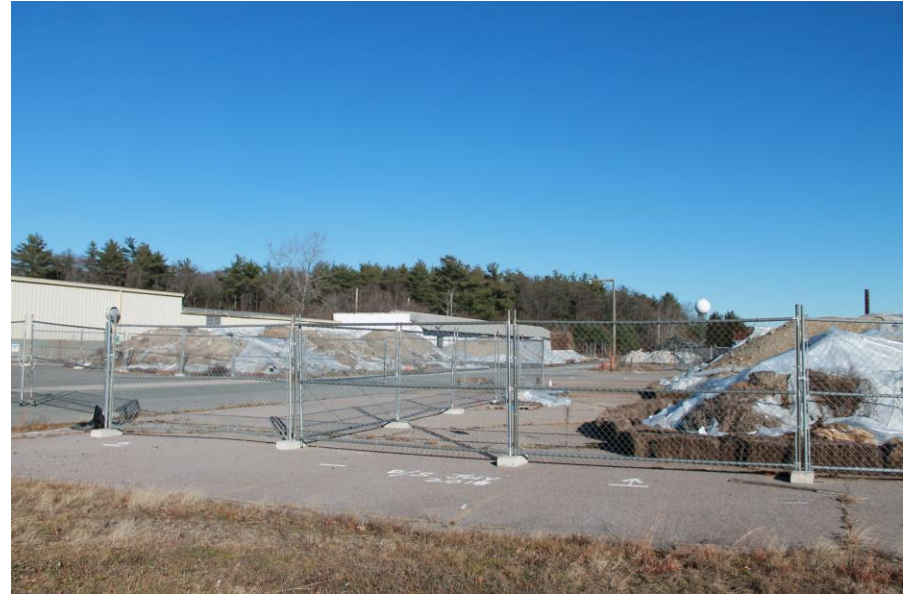
Date: 12/4/2018 Picture No. 10 Location: IOA Comment: Soil piles south of Building 140, looking northeast
