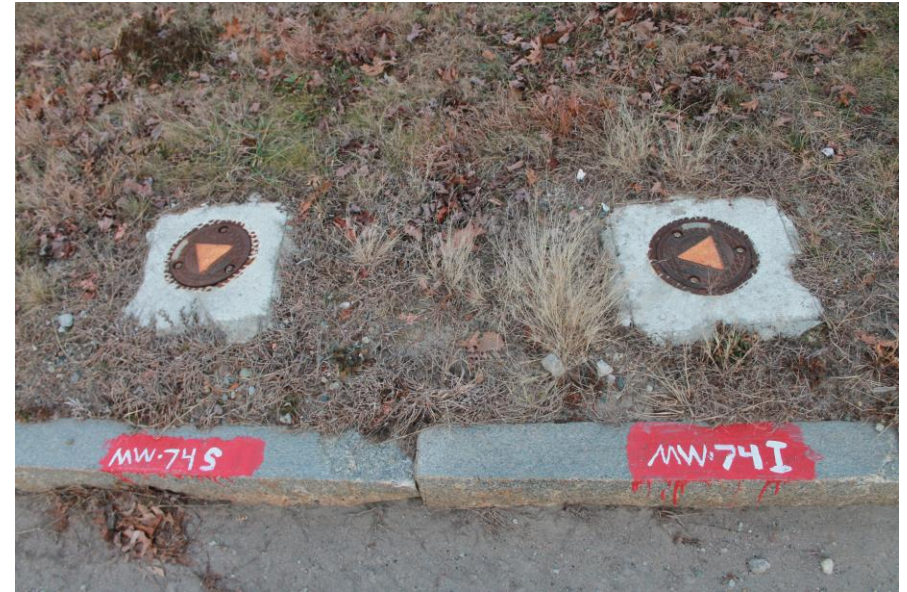
Date: 12/5/2018 Picture No. 18 Location: Building 81 Comment: View of MW-74S and 74I
