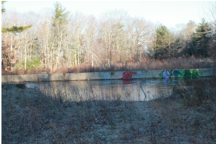
Date: 12/5/2018 Picture No. 7 Location: STP Comment: Former sludge drying bed area, ponded water
