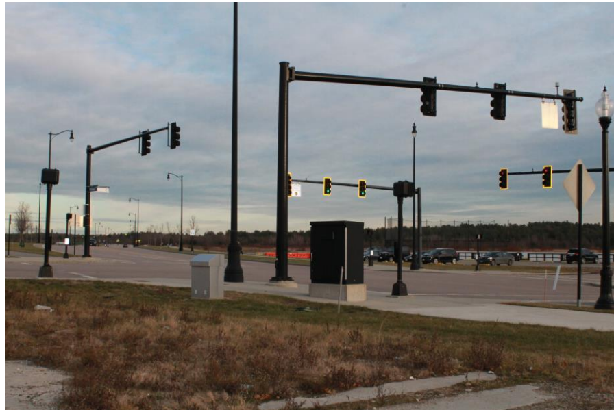
Date: 12/5/2018 Picture No. 3 Location: Hangar 1 Comment: Central portion of Hangar 1 area and intersection of Shea Memorial Dr., Patriot Parkway and Bill Delahunt Parkway
