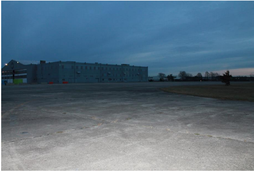
Date: 12/5/2018 Picture No. 17 Location: Building 82 Comment: View of western portion of Building 82 site, looking southeast
