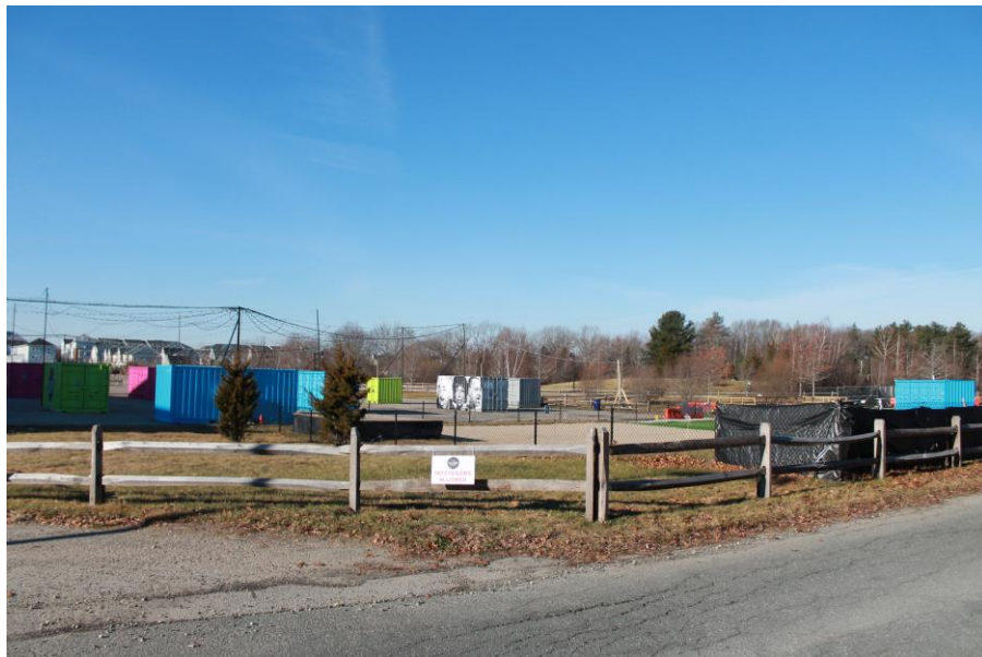
Date: 12/5/2018 Picture No. 11 Location: Building 82 Comment: Northeast portion of site, looking northwest
