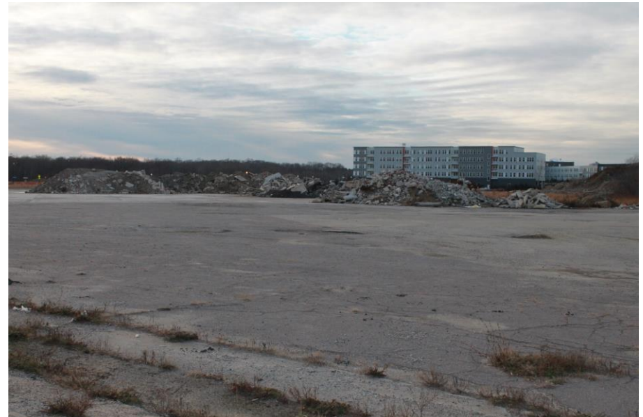
Date: 12/5/2018 Picture No. 4 Location: Hangar 1 Comment: Construction/concrete debris piles located west of AOC Hangar 1
