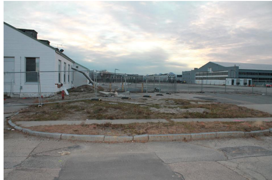
Date: 12/5/2018 Picture No. 12 Location: Building 81 Comment: Demo of Building 11 in progress, looking at northern side of building, facing west
