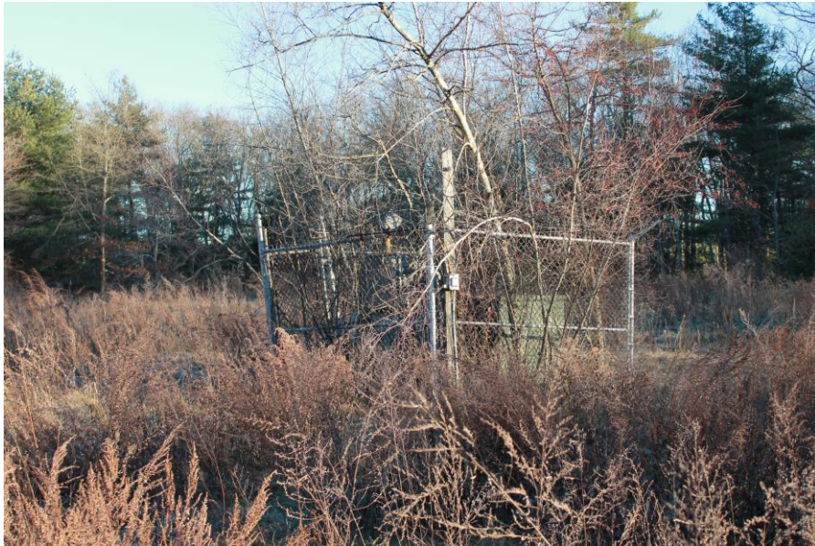
Date: 12/5/2018 Picture No. 5 Location: STP Comment: Chain link fence enclosure around inactive non-PCB transformer
