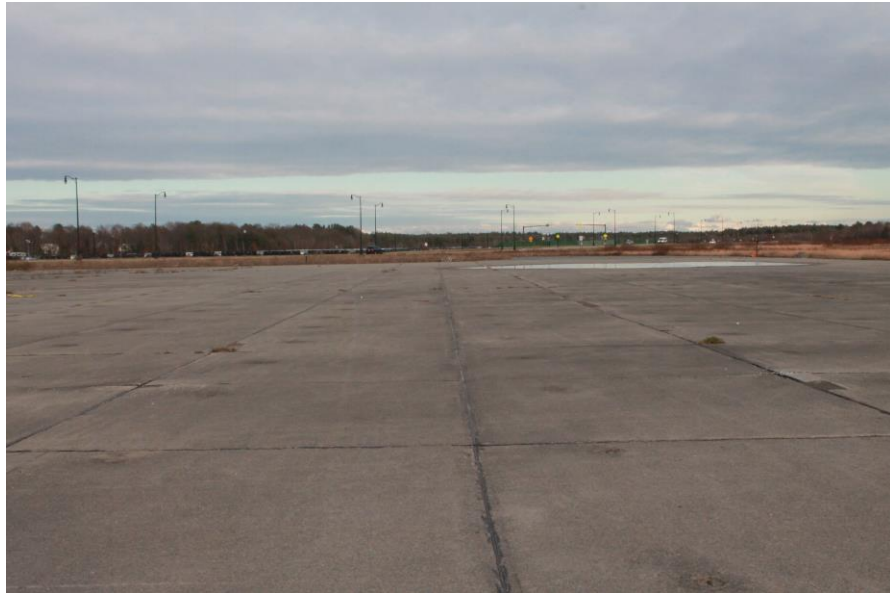
Date: 12/5/2018 Picture No. 5 Location: Hangar 1 Comment: Hangar 1 apron located south of Patriot Parkway, looking toward Bill Delahunt Parkway intersection
