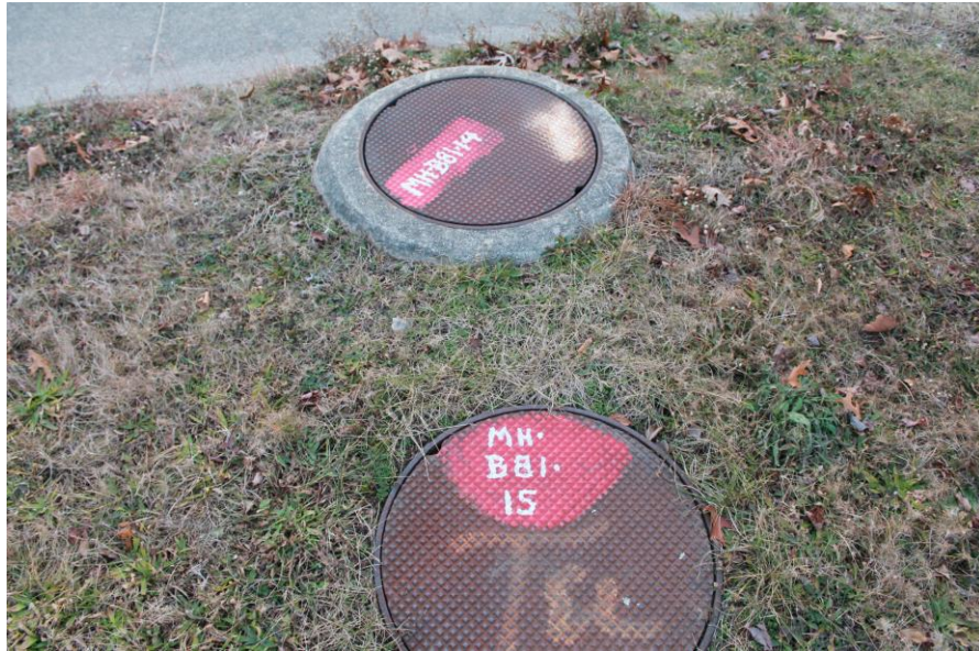
Date: 12/5/2018 Picture No. 17 Location: Building 81 Comment: Manholes B81 14 and 15
