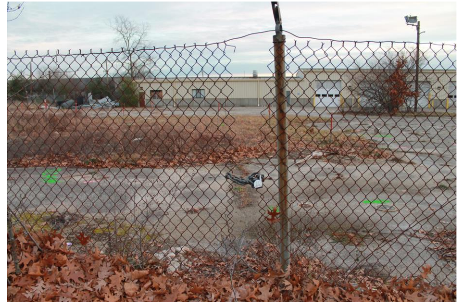
Date: 12/5/2018 Picture No. 10 Location: Building 81 Comment: Cut in fence along northeast portion of site, fence needs permanent repair
