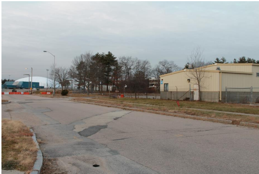
Date: 12/5/2018 Picture No. 3 Location: Building 81 Comment: Building 81 and Building 140 looking north up Shea Memorial Dr.
