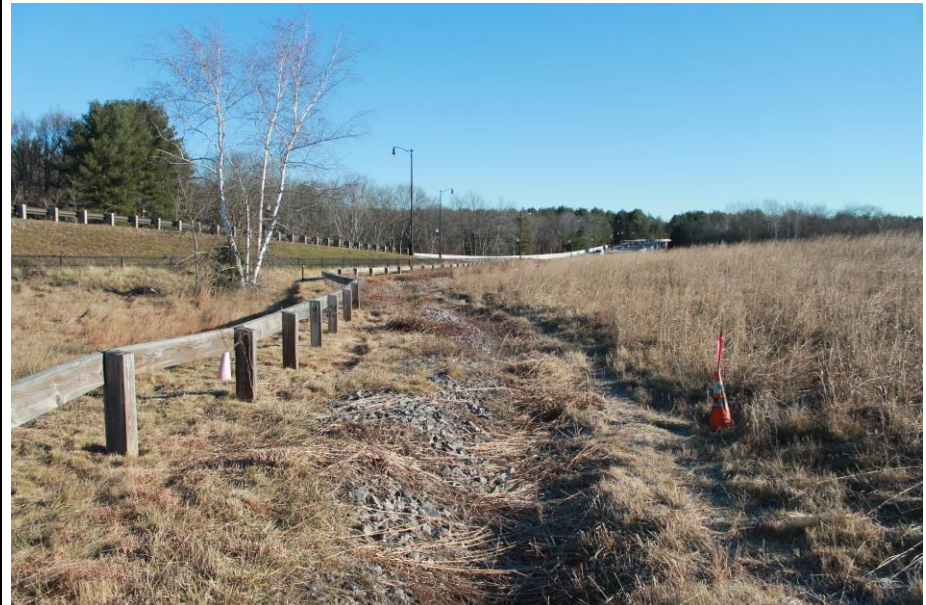
Date: 12/5/2018 Picture No. 20 Location: RDA Comment: Wood guard rail and riprap drainage ditch along northern perimeter of RDA
