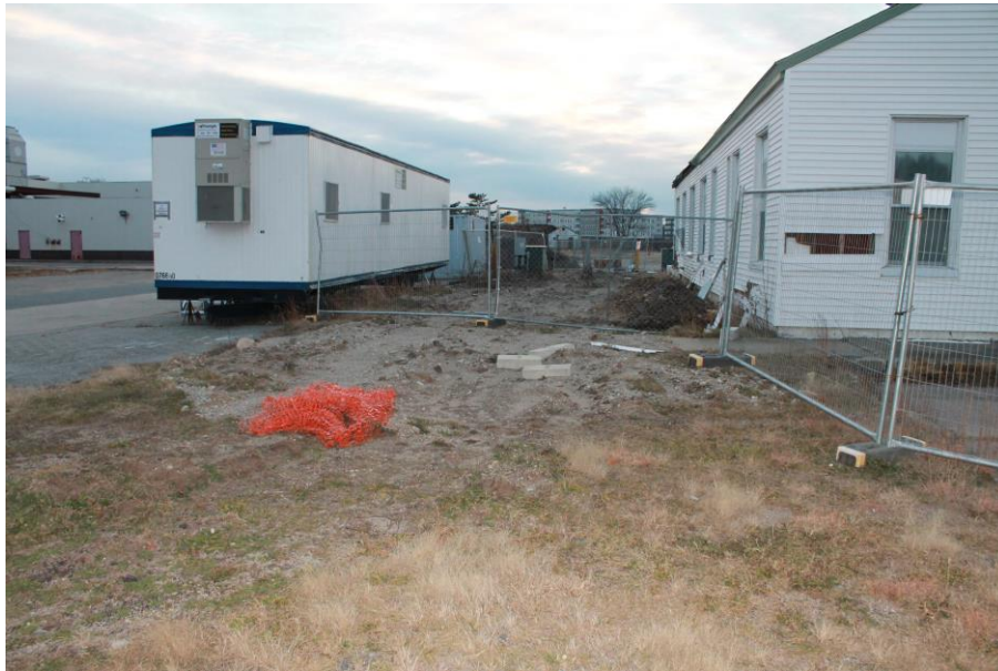
Date: 12/5/2018 Picture No. 11 Location: Building 81 Comment: Demo of Building 11 in progress, area fenced, looking at southern side of Building 11
