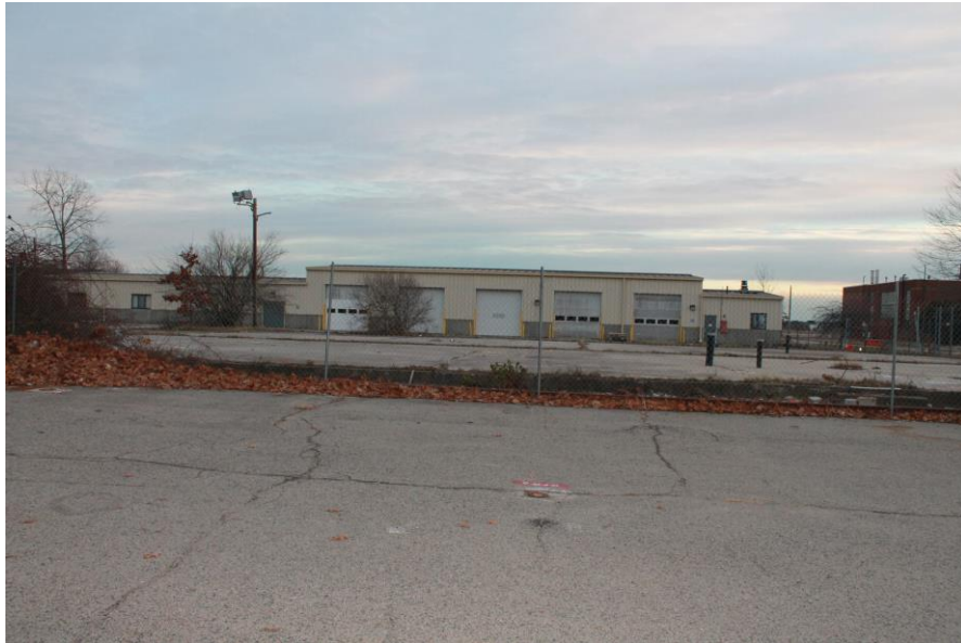
Date: 12/5/2018 Picture No. 5 Location: Building 81 Comment: Building 81 area, looking south from Redfield Rd.
