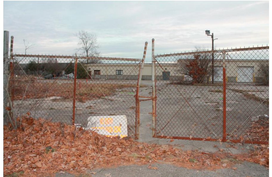
Date: 12/5/2018 Picture No. 2 Location: Building 81 Comment: Building 81 access gate located on north side of site
