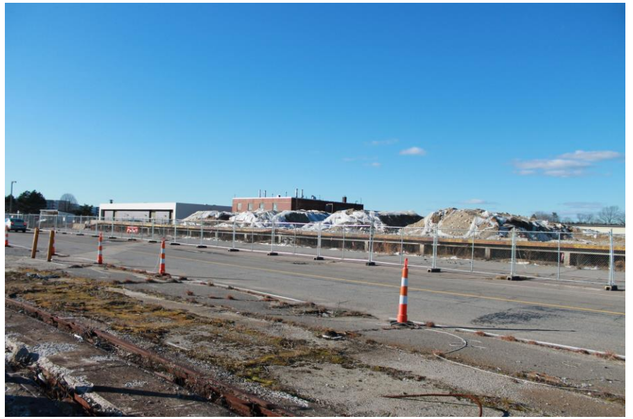
Date: 12/4/2018 Picture No. 12 Location: IOA Comment: Soil piles, looking northwest from Cummings Rd.
