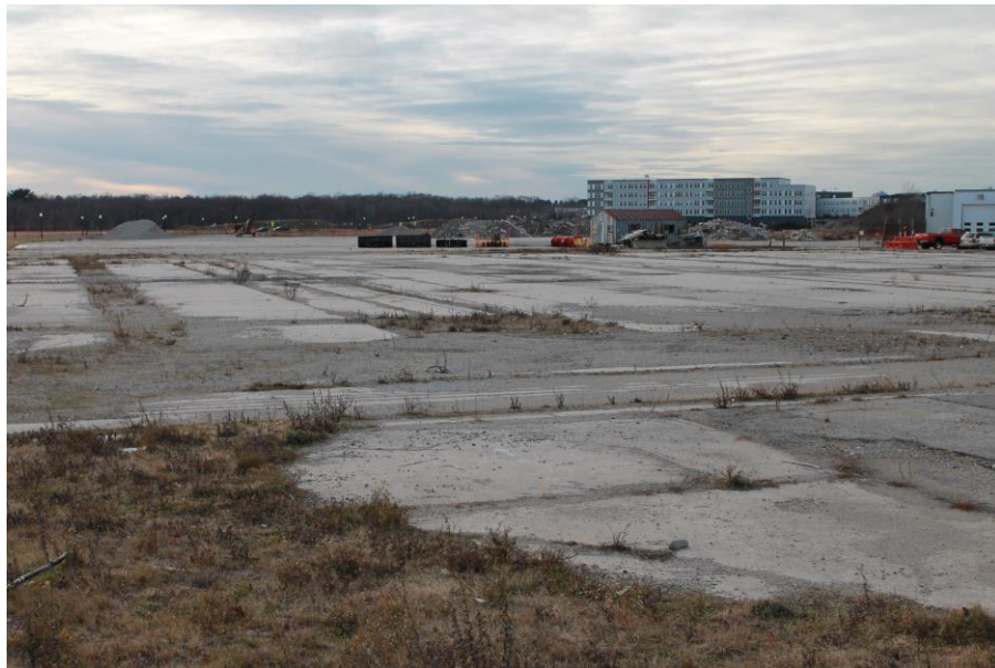
Date: 12/5/2018 Picture No. 7 Location: Hangar 1 Comment: Location of former Hangar 1, looking west
