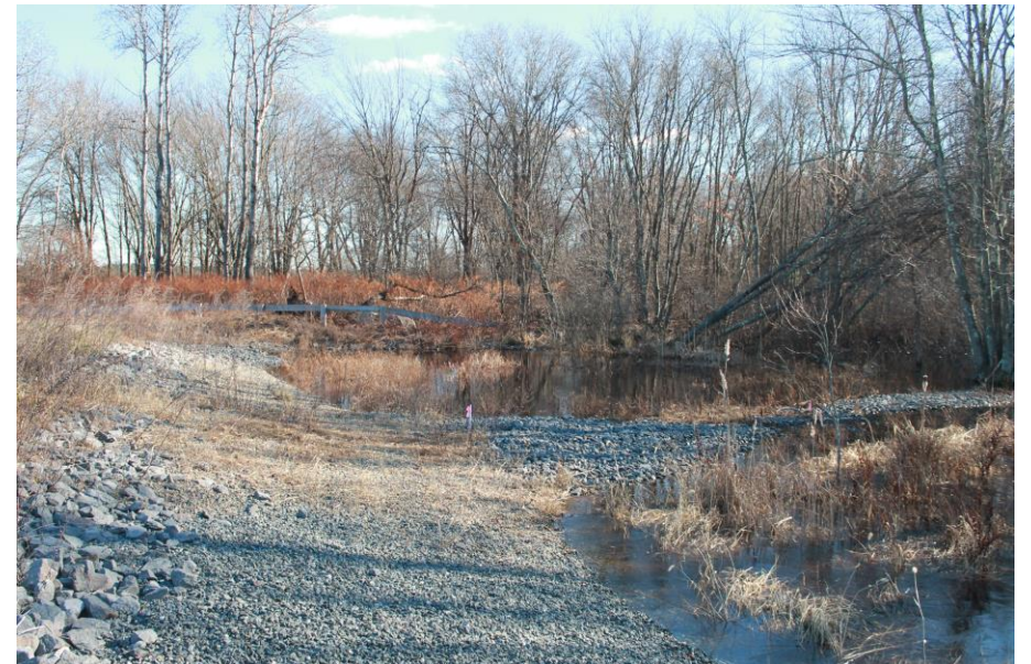
Date: 12/4/2018 Picture No. 16 Location: WGL Comment: View of South Level Spreader, high surface water levels
