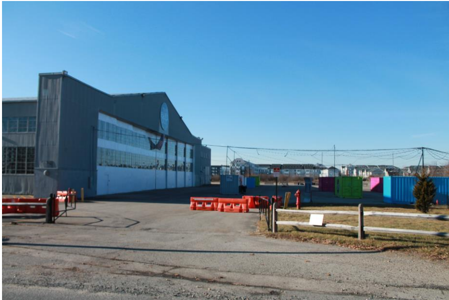
Date: 12/5/2018 Picture No. 13 Location: Building 82
