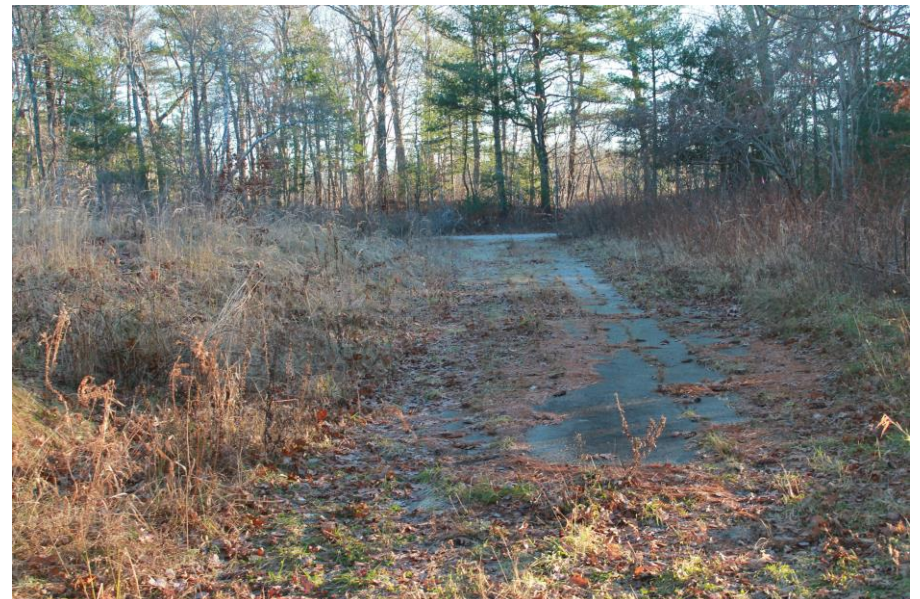
Date: 12/5/2018 Picture No. 4 Location: STP Comment: Access road located south of former sludge drying bed area
