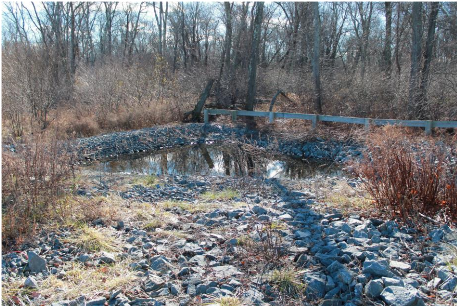
Date: 12/4/2018 Picture No. 11 Location: WGL Comment: View of North Level Spreader
