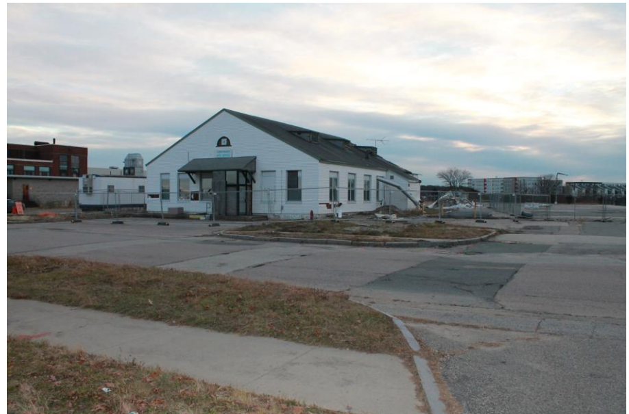
Date: 12/5/2018 Picture No. 16 Location: Building 81 Comment: View of Building 11, partially demolished
