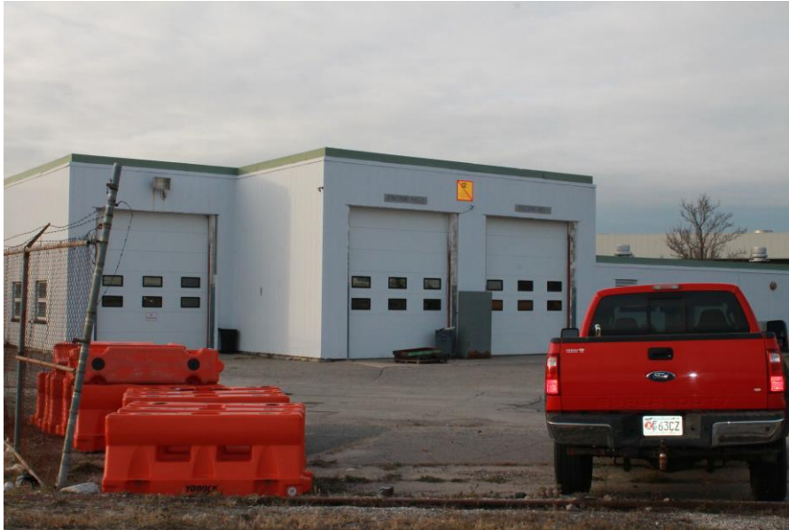
Date: 12/4/2018 Picture No. 1 Location: IOA Comment: Building 96 located within the IOA area
