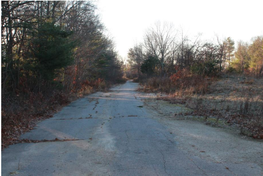
Date: 12/5/2018 Picture No. 1 Location: STP Comment: Access road to STP, looking south
