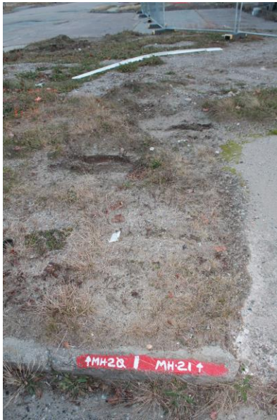
Date: 12/5/2018 Picture No. 9 Location: Building 81 Comment: Could not locate manholes MH-20 and MH-21, may be covered with soil from demo of Building 11
