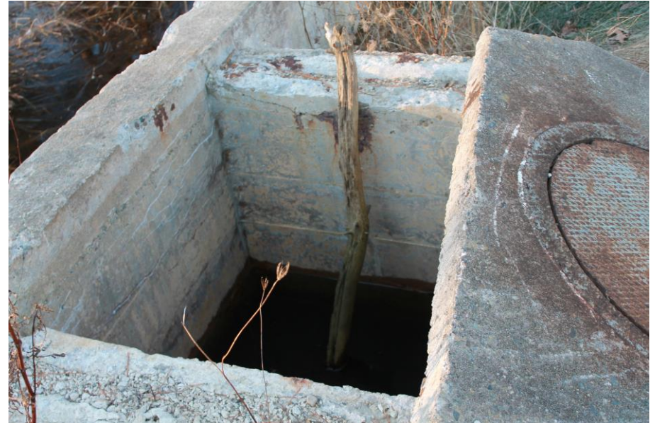
Date: 12/5/2018 Picture No. 10 Location: STP Comment: Manhole structure associated with former sludge drying beds
