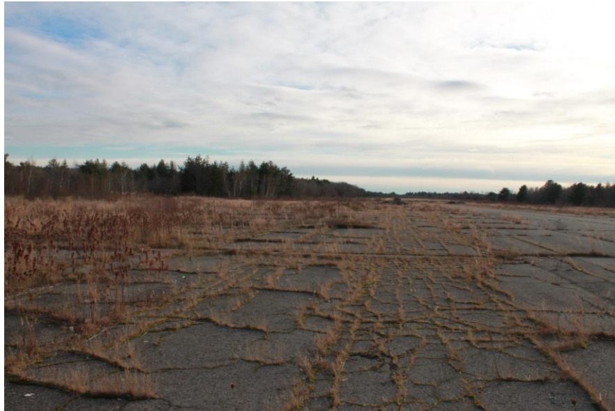
Date: 12/5/2018 Picture No. 1 Location: FFTA Comment: Central portion of FFTA, looking south
