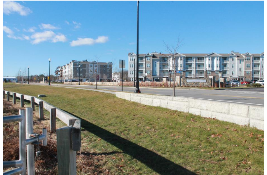
Date: 12/4/2018 Picture No. 2 Location: WGL
