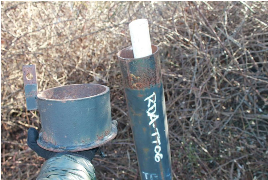
Date: 12/5/2018 Picture No. 15 Location: RDA Comment: TT-06 well casing cover cannot be secured, PVC needs to be trimmed
