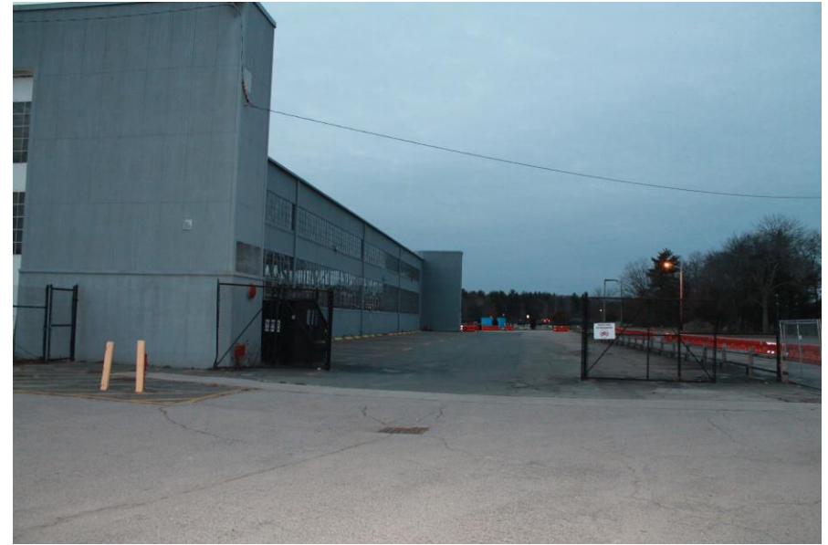
Date: 12/5/2018 Picture No. 2 Location: Building 82 Comment: Eastern portion of Building 82 area looking north
