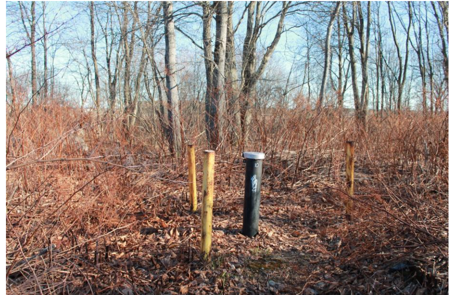
Date: 12/4/2018 Picture No. 6 Location: WGL Comment: LFG-10 cap not secured to casing
