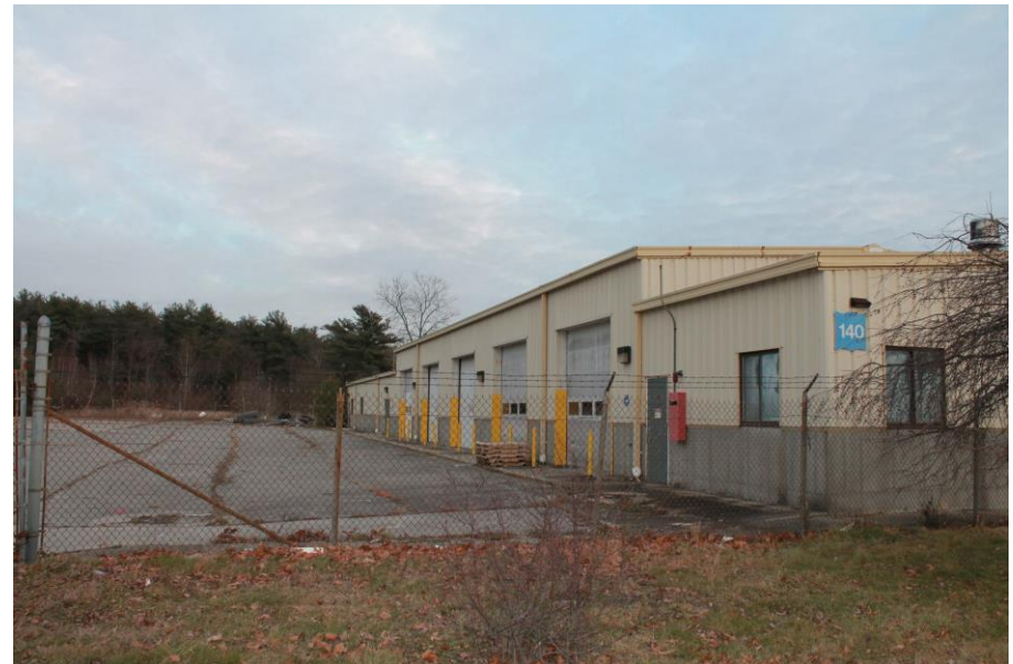
Date: 12/5/2018 Picture No. 4 Location: Building 81 Comment: Building 81 and Building 140, looking east
