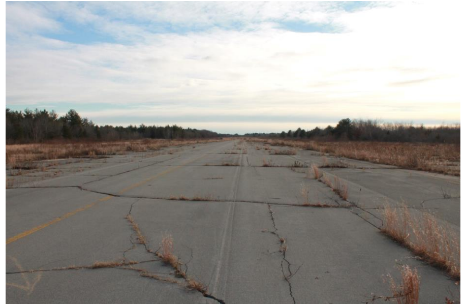
Date: 12/5/2018 Picture No. 6 Location: FFTA Comment: Looking south across FFTA
