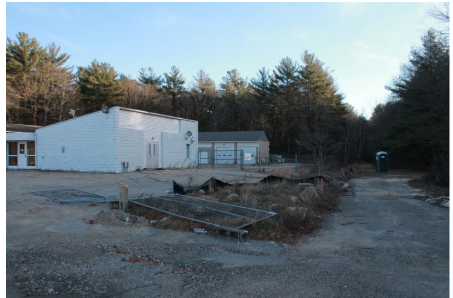
Date: 12/6/2018 Picture No. 14 Location: SRA Comment: Northern access path to SRA
