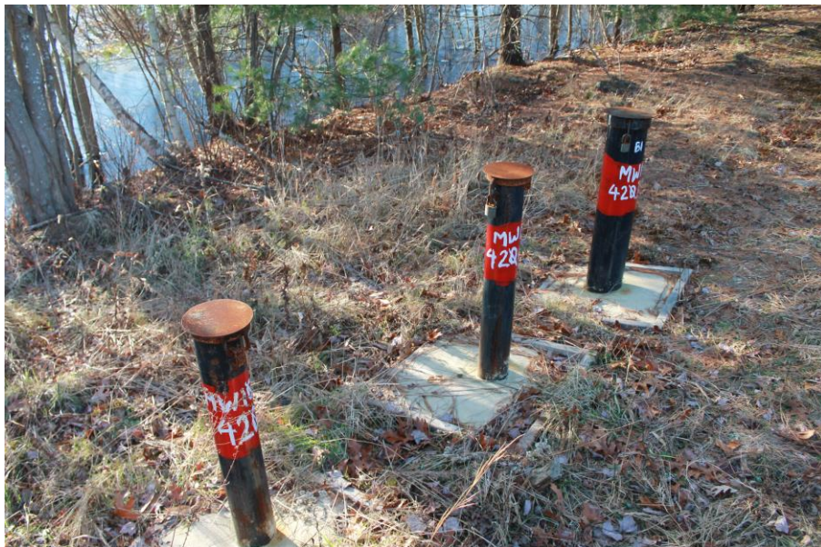
Date: 12/6/2018 Picture No. 11 Location: SRA Comment: MW420S, BR1 and BR2 located in south-central portion of site
