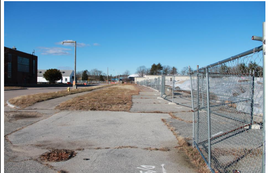
Date: 12/4/2018 Picture No. 4 Location: IOA Comment: Construction fence along western perimeter of IOA excavation
