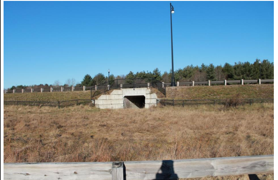
Date: 12/5/2018 Picture No. 16 Location: RDA Comment: Turtle bridge located north of RDA
