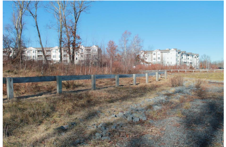
Date: 12/4/2018 Picture No. 26 Location: WGL Comment: View of western access road and riprap, looking northeast
