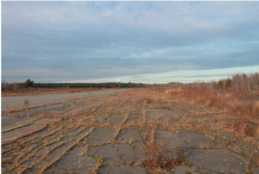
Date: 12/5/2018 Picture No. 5 Location: FFTA Comment: Looking north from site up Taxiway
