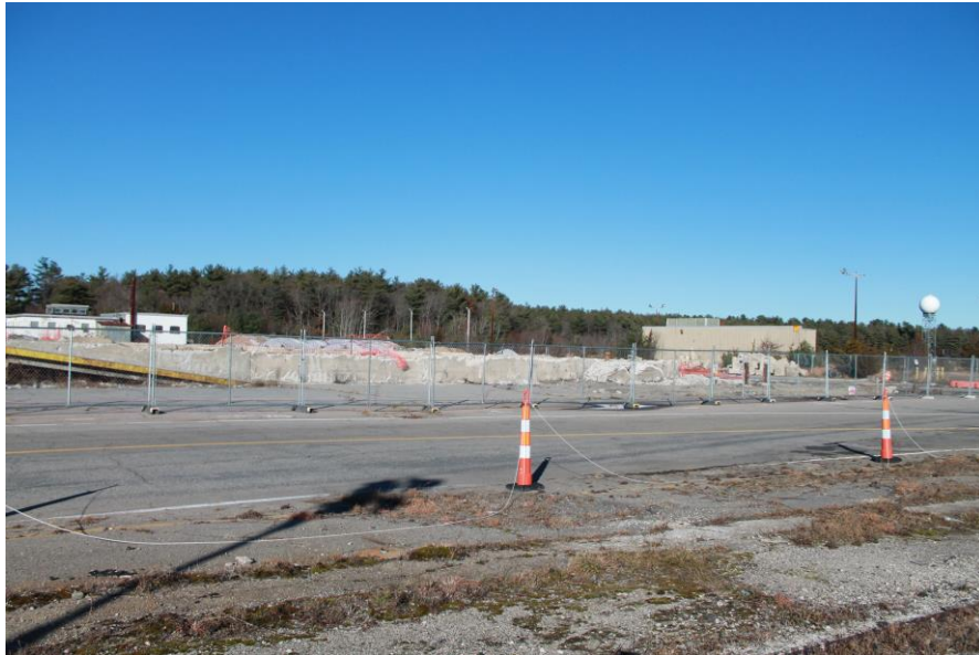
Date: 12/4/2018 Picture No. 17 Location: IOA Comment: View of eastern portion of IOA excavation, looking northeast from Cummings Dr.
