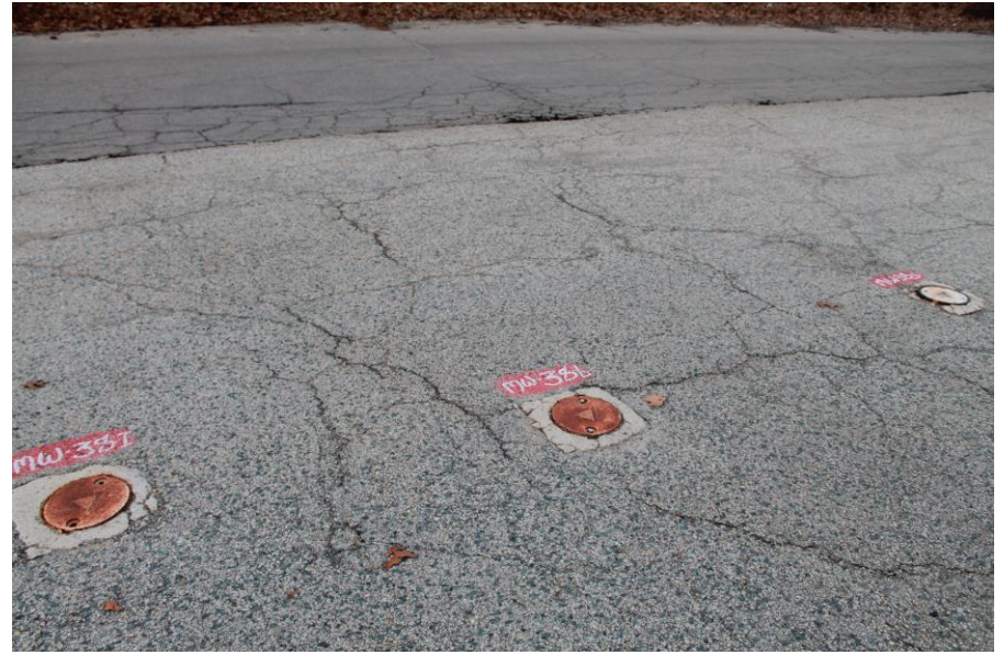
Date: 12/5/2018 Picture No. 14 Location: Building 81 Comment: MW381, 38B, and 38S monitoring wells located in northern portion of site
