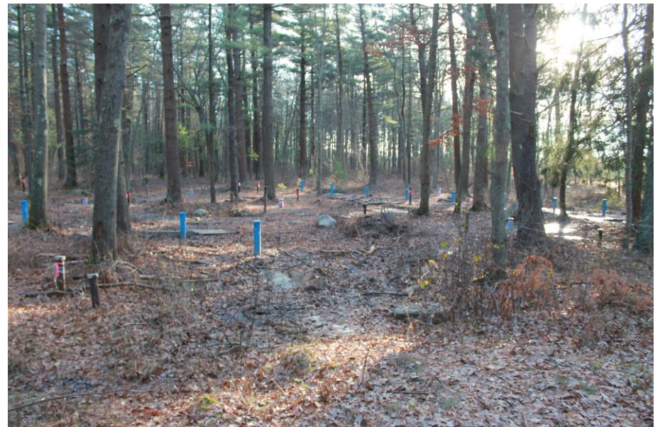
Date: 12/6/2018 Picture No. 12 Location: SRA Comment: Newly installed weathered bedrock injection wells Eastern Weathered Bedrock Treatment Area and PRB2
