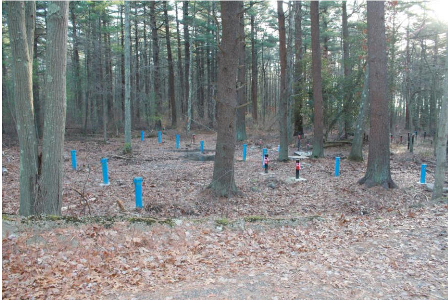
Date: 12/6/2018 Picture No. 13 Location: SRA Comment: Newly installed weathered bedrock injection wells located north of Overburden TTZ, PRB1
