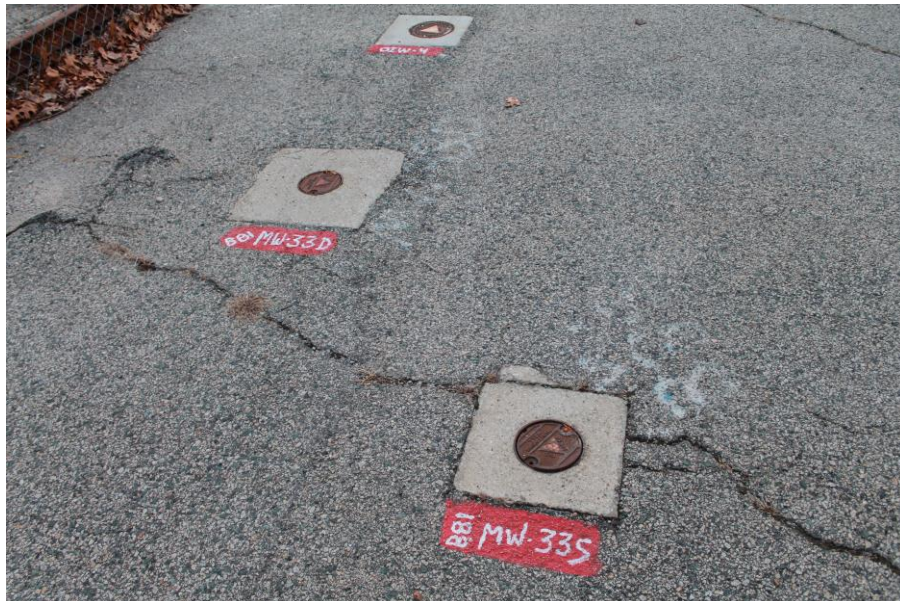
Date: 12/5/2018 Picture No. 7 Location: Building 81 Comment: Building 81, Monitoring wells MW33S and 33D located in northern portion of site
