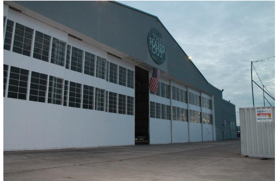
Date: 12/5/2018 Picture No. 6 Location: Building 82 Comment: Hangar 2 current use includes storage of cars/vehicles and event venue for concerts in summer
