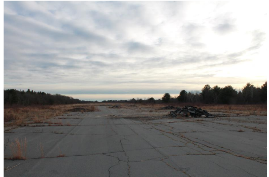
Date: 12/5/2018 Picture No. 10 Location: FFTA Comment: Test pits located south of FFTA LUC area
