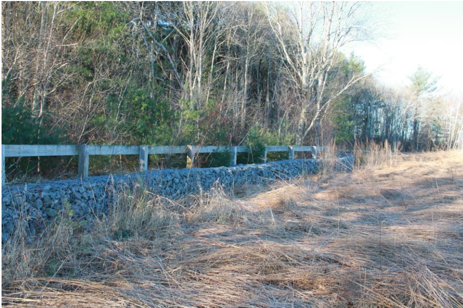
Date: 12/5/2018 Picture No. 3 Location: RDA
