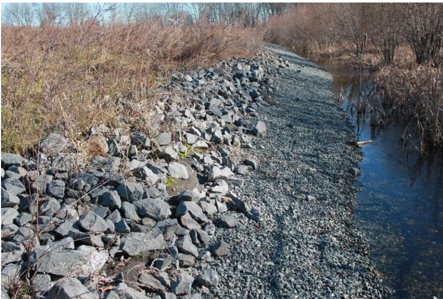
Date: 12/4/2018 Picture No. 7 Location: WGL Comment: Minor erosion of riprap and exposed geotextile observed along southern perimeter of WGL
