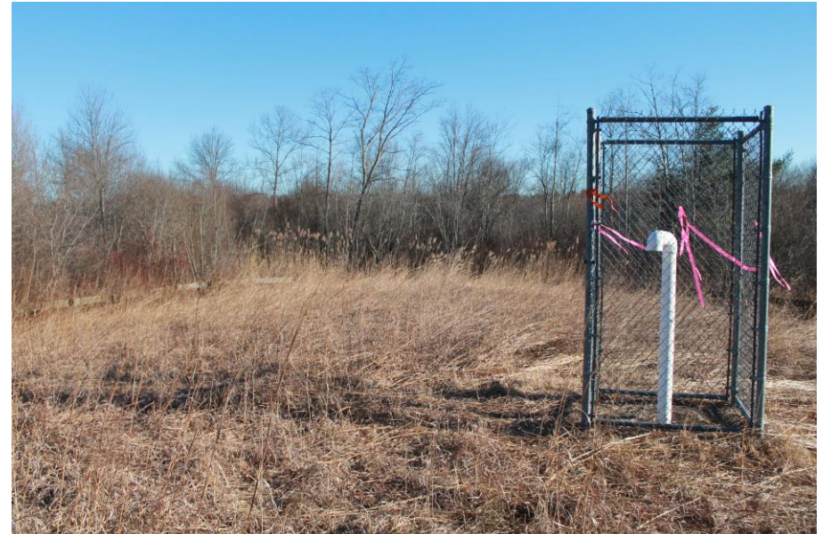
Date: 12/5/2018 Picture No. 4 Location: RDA
