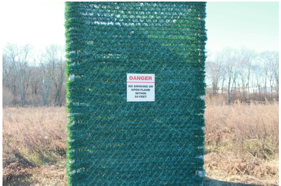
Date: 12/4/2018 Picture No. 4 Location: WGL
