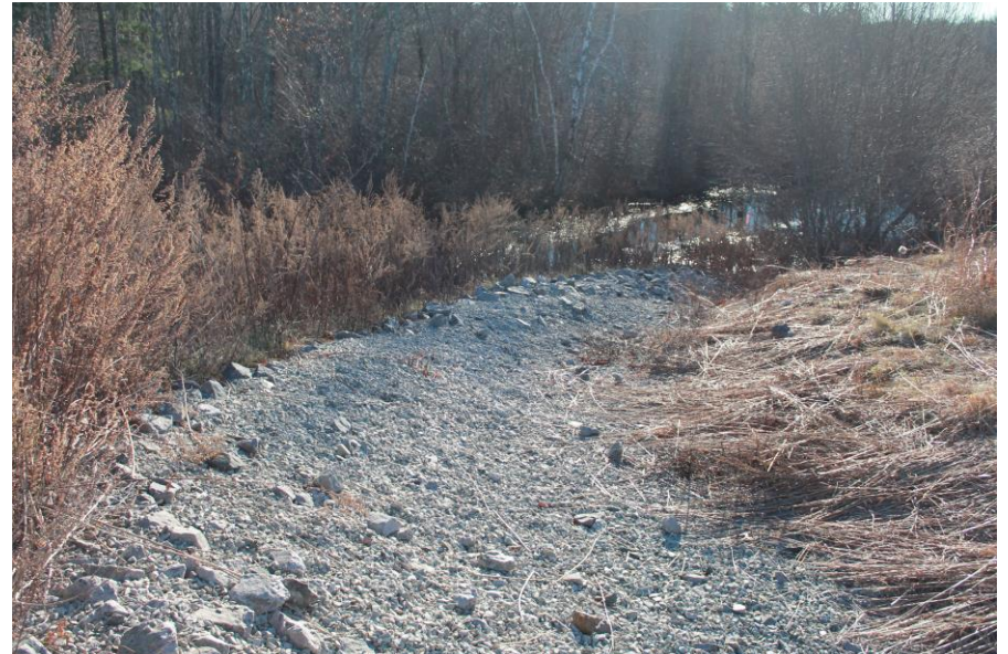
Date: 12/5/2018 Picture No. 10 Location: RDA Comment: Riprap drainage swale in northeast corner of RDA, looking south
