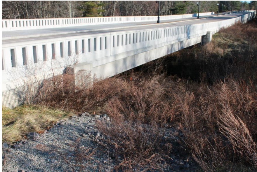
Date: 12/5/2018 Picture No. 1 Location: RDA
