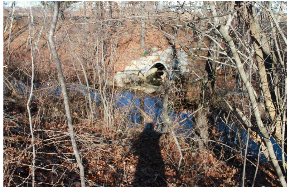
Date: 12/4/2018 Picture No. 24 Location: WGL
