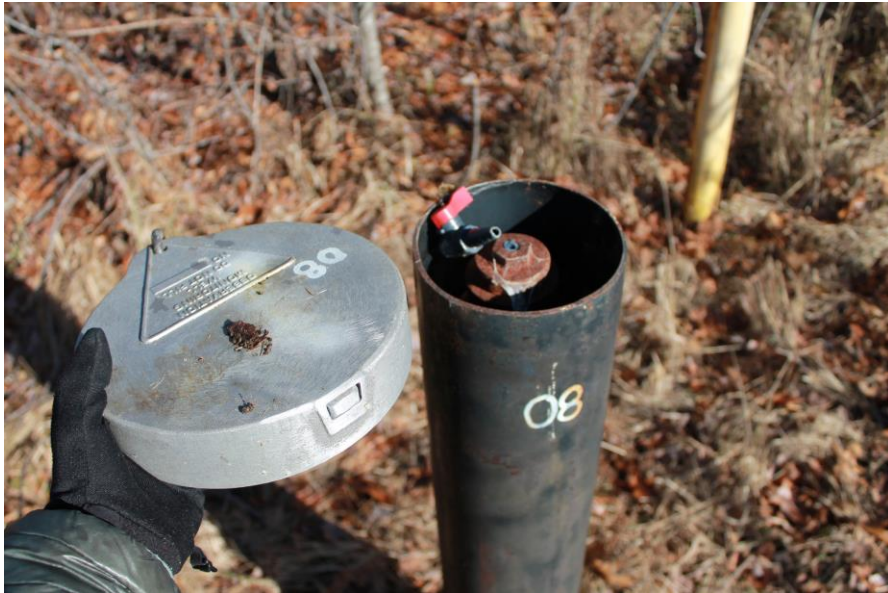
Date: 12/4/2018 Picture No. 5 Location: WGL Comment: LFG-08 cannot lock, needs to be modified so top sits flush with casing
