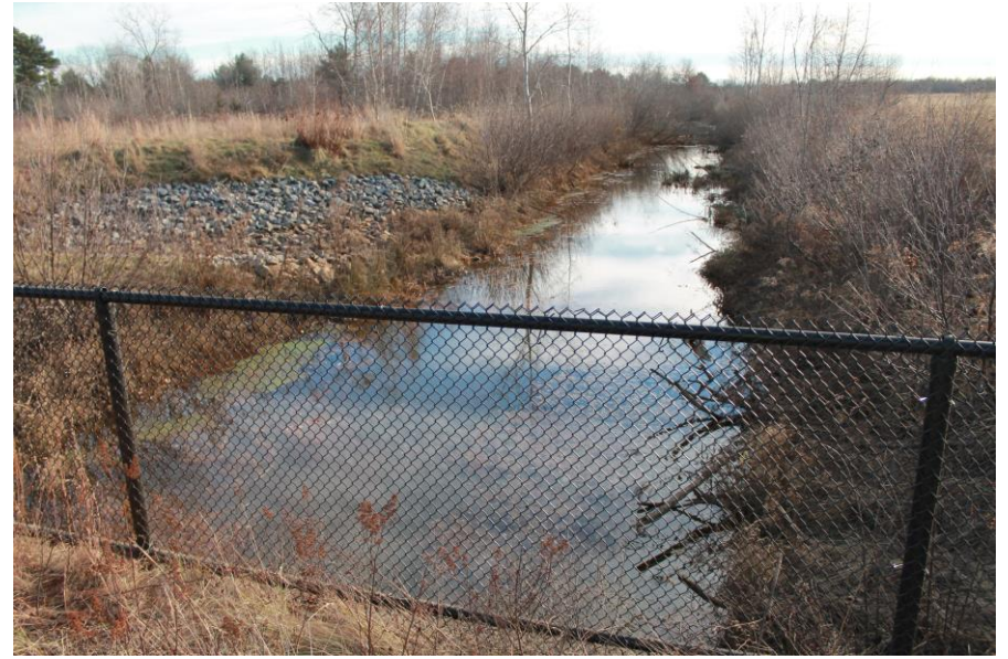
Date: 12/5/2018 Picture No. 14 Location: Hangar 1 Comment: TACAN Outfall, looking southwest
