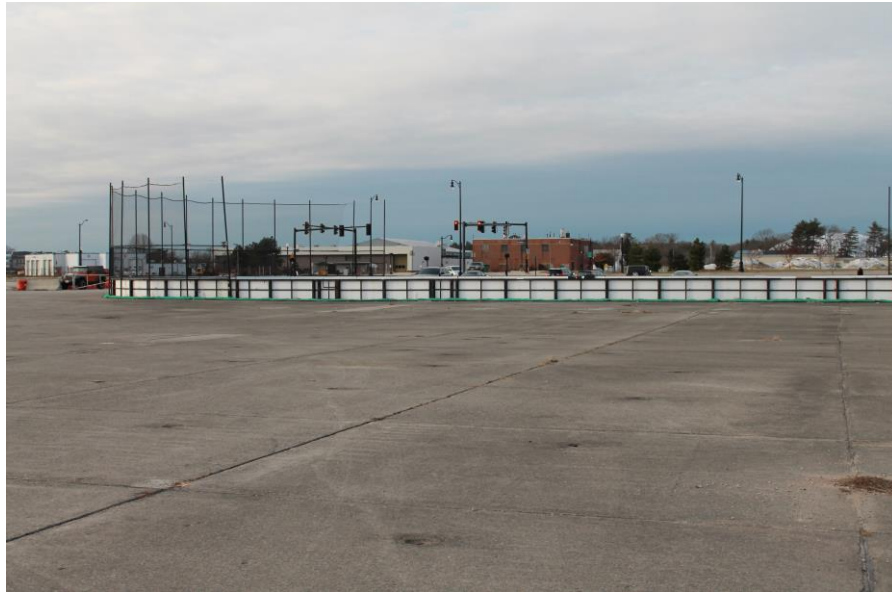
Date: 12/5/2018 Picture No. 17 Location: Hangar 1 Comment: View of ice rink and intersection of Shea Memorial Dr. and Bill Delahunt and Patriot Parkway
