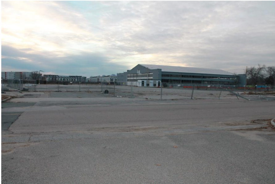
Date: 12/5/2018 Picture No. 1 Location: Building 81 Comment: Area west of Building 81, looking west toward Building 82
