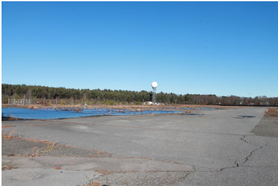
Date: 12/4/2018 Picture No. 3 Location: IOA Comment: East mat ditch, looking northeast
