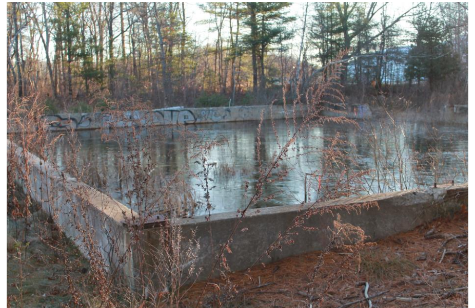
Date: 12/5/2018 Picture No. 8 Location: STP Comment: Historic location of sludge drying beds
