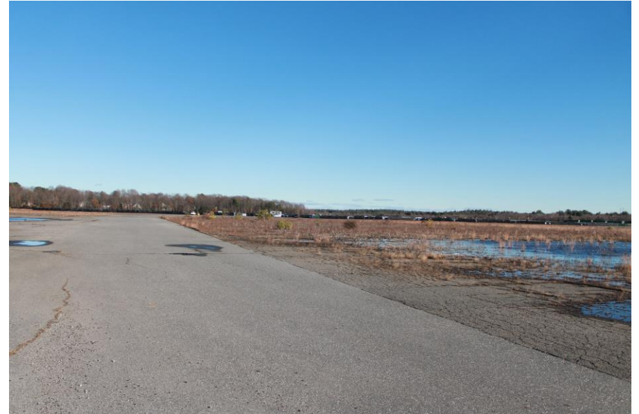
Date: 12/4/2018 Picture No. 2 Location: IOA Comment: East mat ditch, looking east
