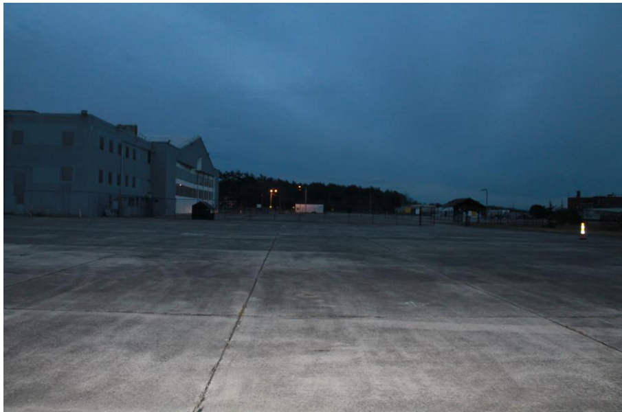
Date: 12/5/2018 Picture No. 16 Location: Building 82
