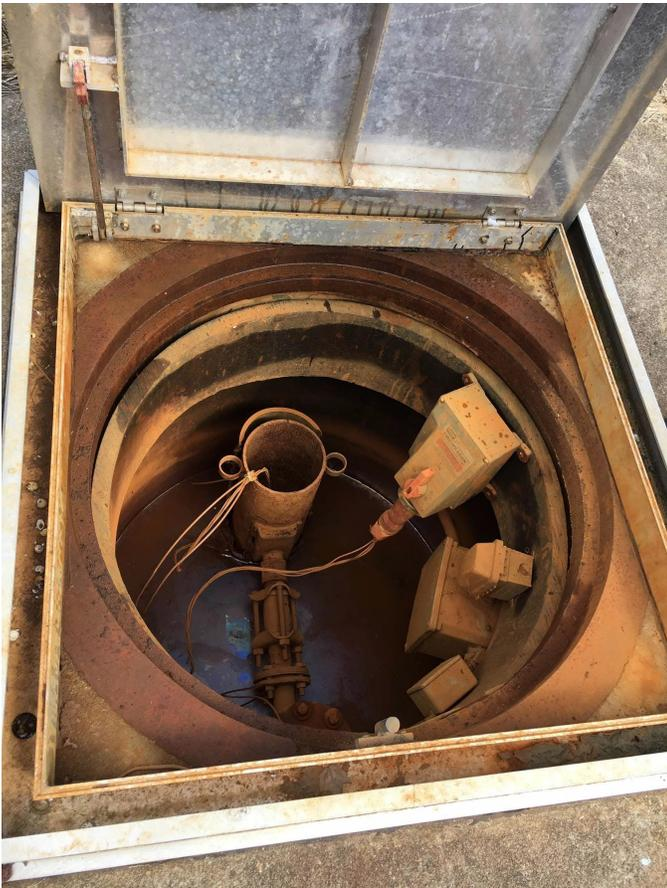
16. EW-7 retrofitted with pitless adapter installed to allow for eased redevelopment
