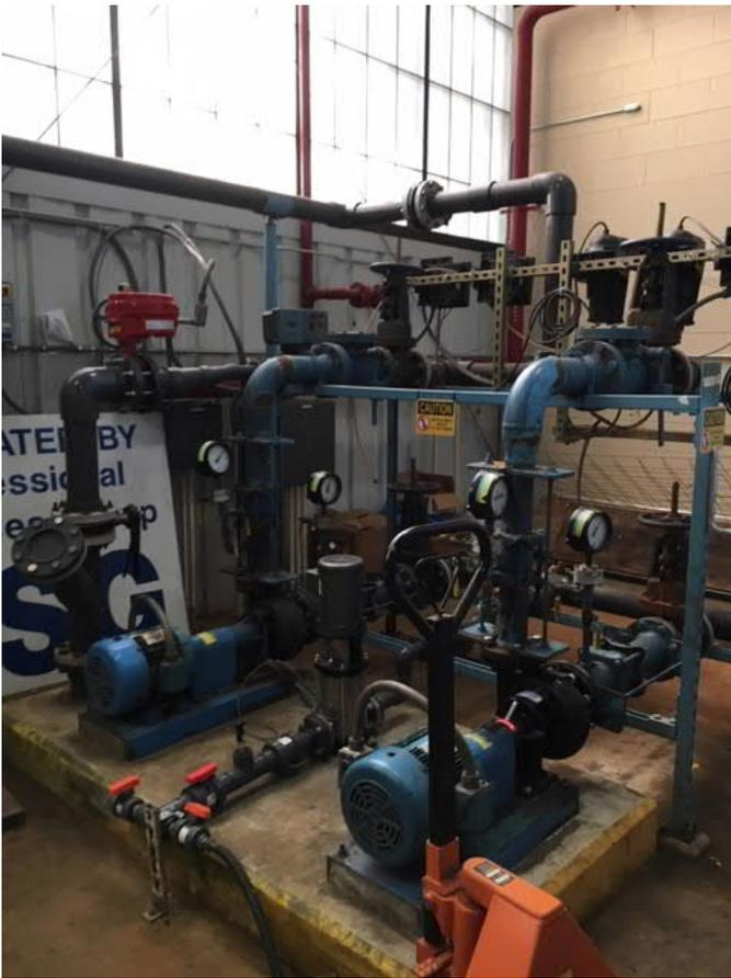
5. Pumps and new piping from Effluent Holding Tank T-17 configured to recycle treated effluent for reuse as process water
