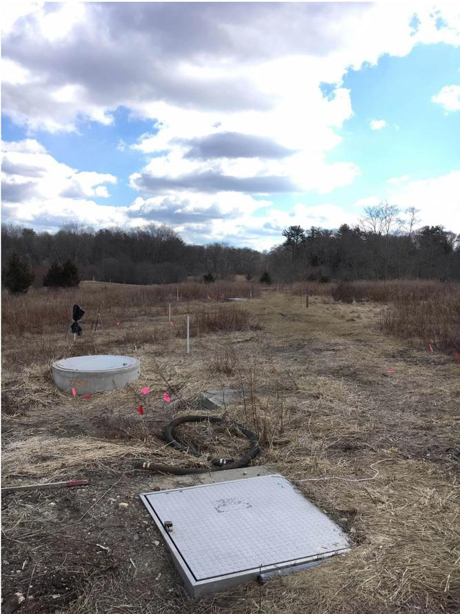
14. Extraction well EW-6a (installed in 2015 to replace EW-6). White posts in background were installed for the Parsons study
