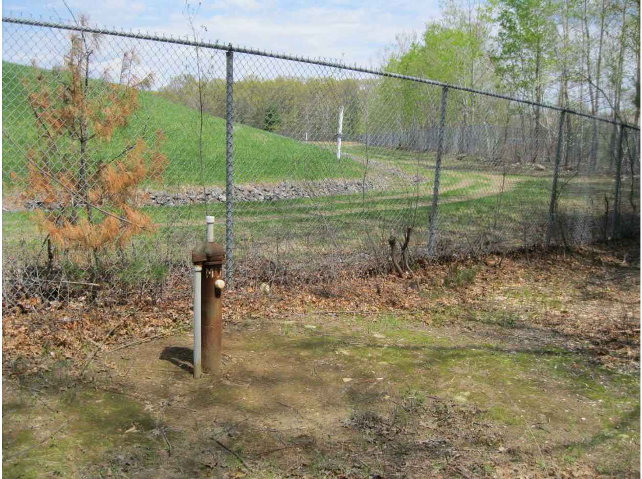
Photo #2. Extraction Well MLF, just outside fence that surrounds Industrial Landfill (gate in fence for access to well is about 40 feet to the left). May 7, 2019.
