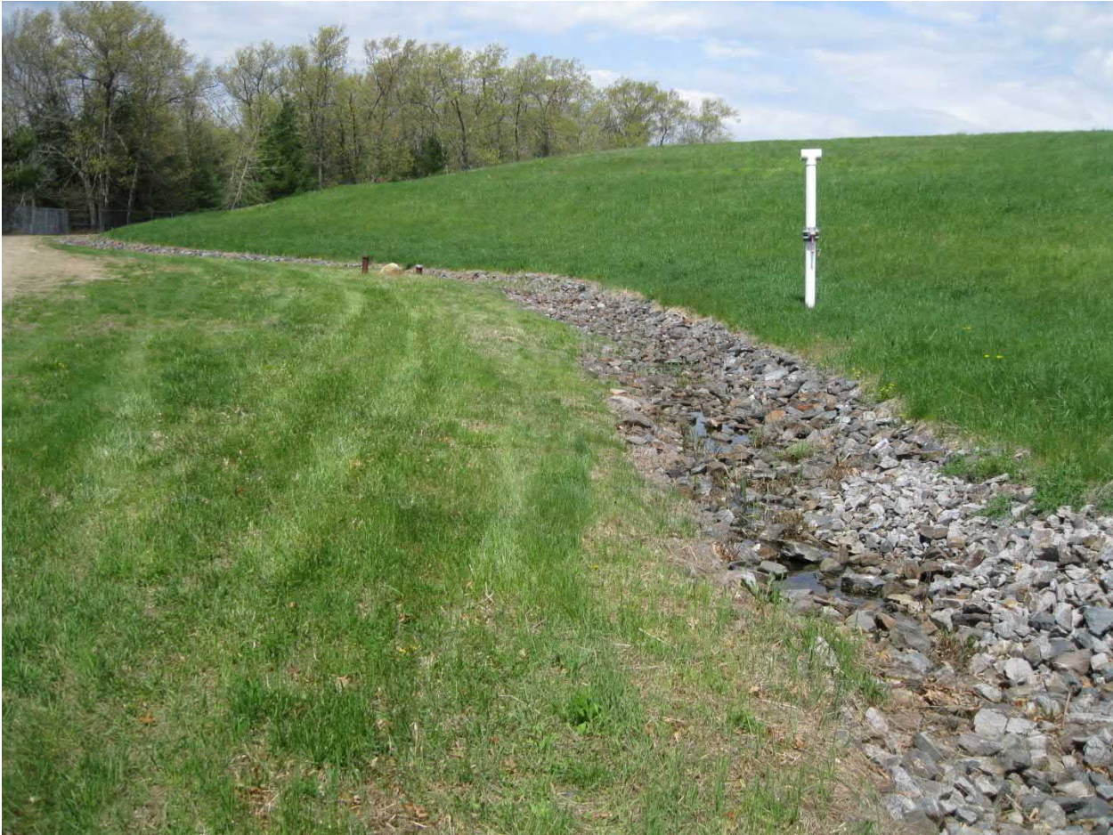
Photo #1. Perimeter drain on south side of Industrial Landfill. Note general lack of vegetation in rip rap, open gas vent, and healthy appearance of grass cover on landfill. May 7, 2019
