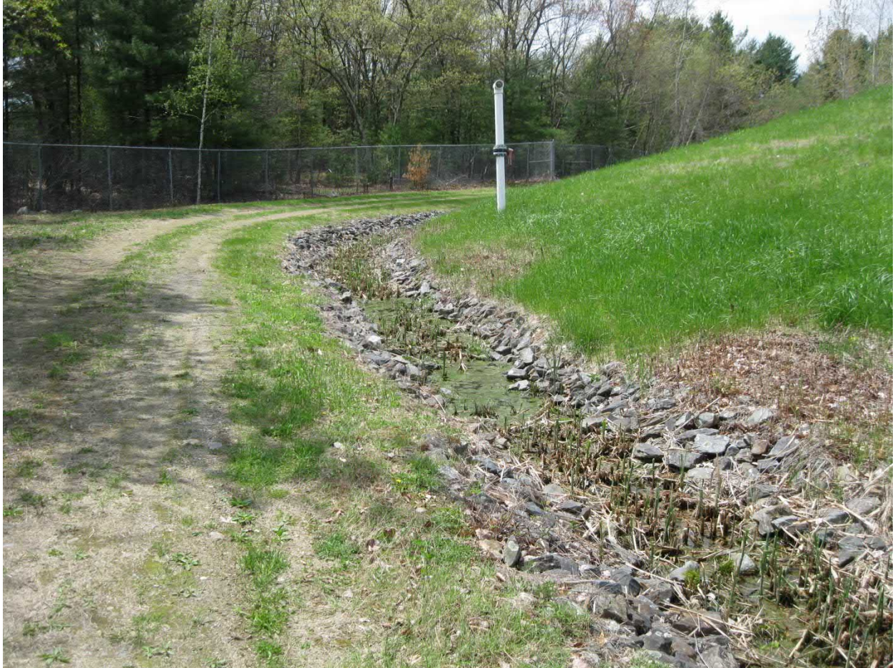
Photo #3. Perimeter drain on southeast side of Industrial Landfill. Note vegetation and water in rip rap channel, landfill perimeter fence, and open gas vent. May 7, 2019
