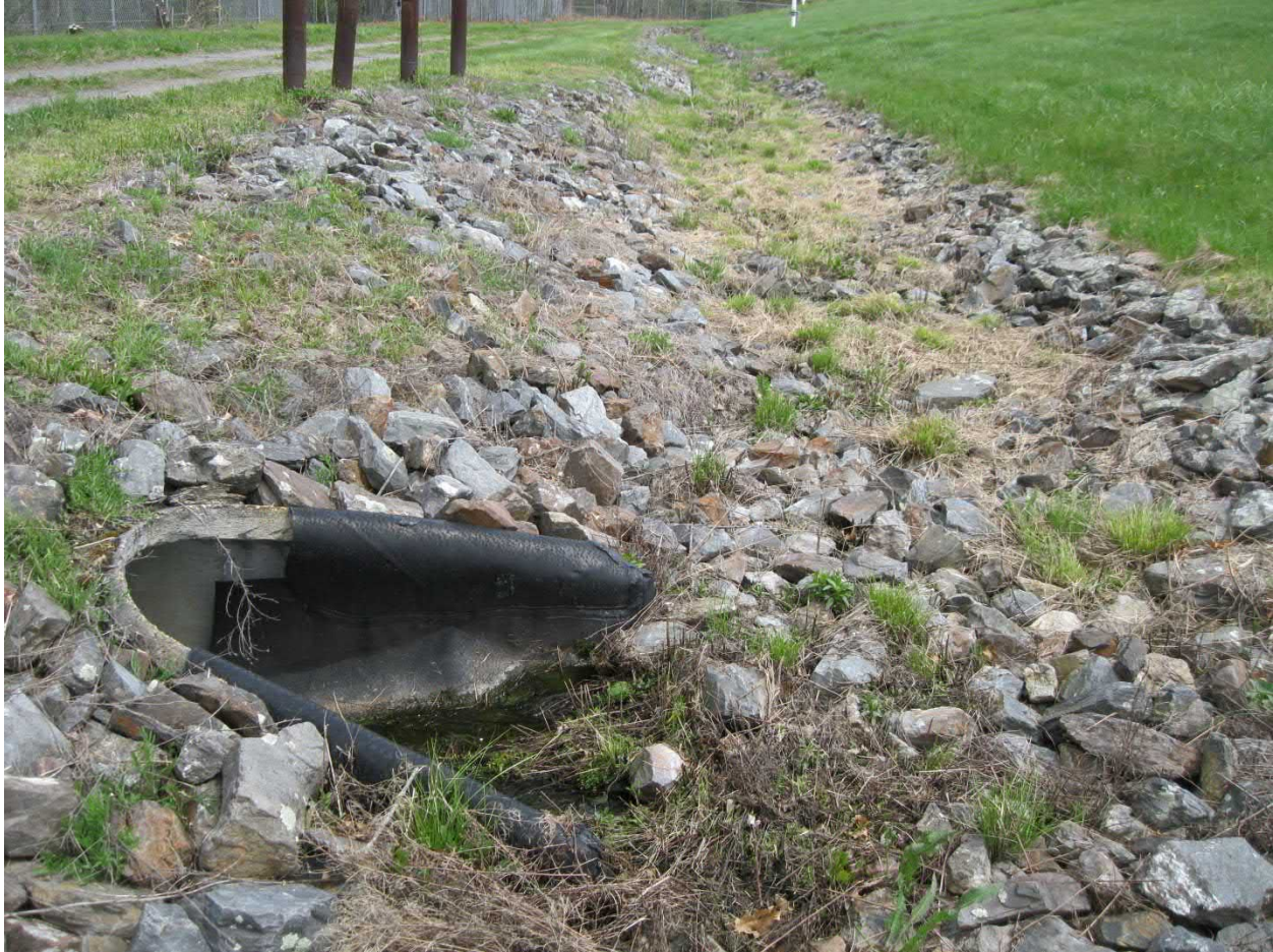
Photo #4. Water draining (despite vegetation) from perimeter drainage channel into culvert, that conveys water beneath perimeter roadway and fence to low area on north side of landfill. Note protective pipes on monitoring wells (4 wells) of LF-11 cluster. May 7, 2019.
