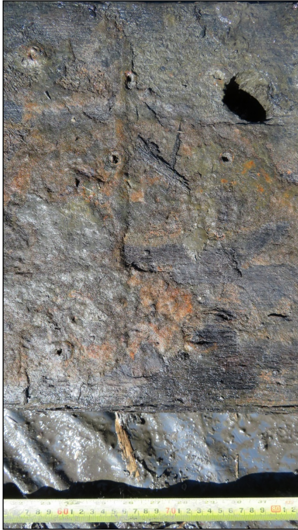
Figure 21. Tarred animal hair “felting” and sheathing nail holes on the exterior surfaces of NBHSS UAD SW#3’s hull planking and keel provided evidence that the vessel’s hull had once been sheathed in protective sacrificial wooden hull sheathing (photographs by David Robinson, DSRA).
