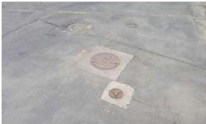
Photo 6. Monitoring wells RW-2R, RW-6, RW-2RA
