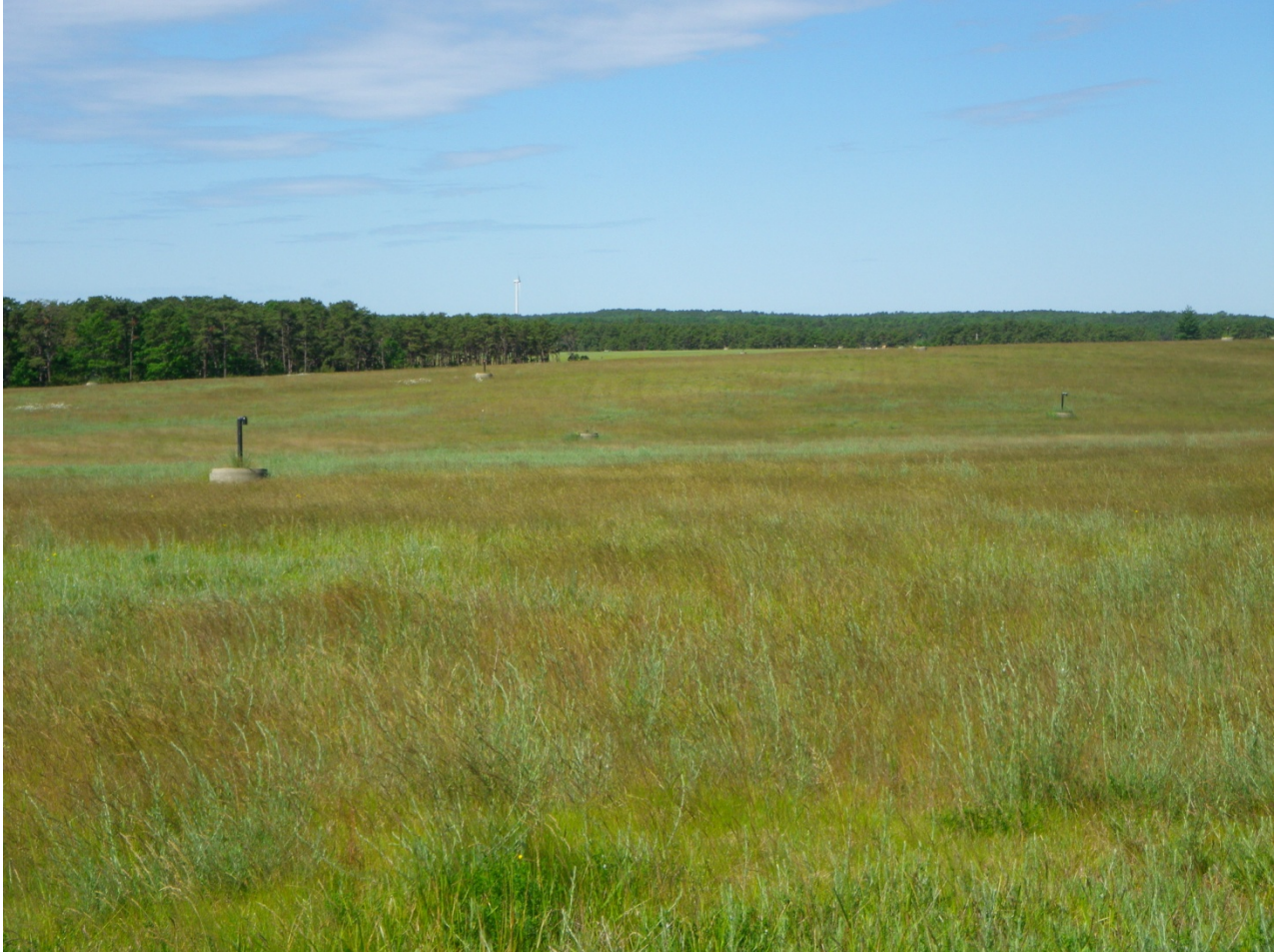
LF-1 Photo 5: LF-1 landfill cap
