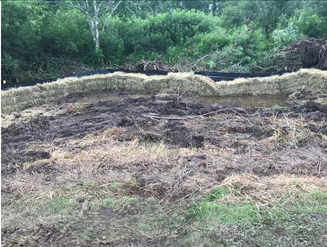
Silt fence and hay bale installation - MW-1.
