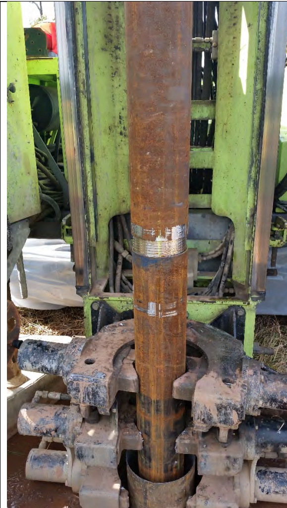
Installing permanent 6-inch casing – MW-10.
