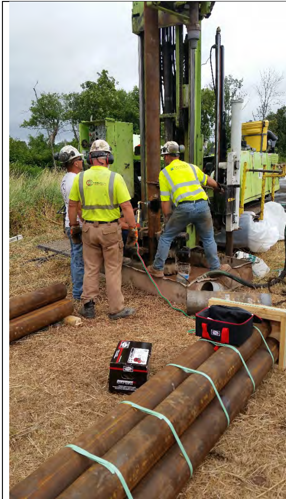
Installing permanent 6-inch casing – MW-10.
