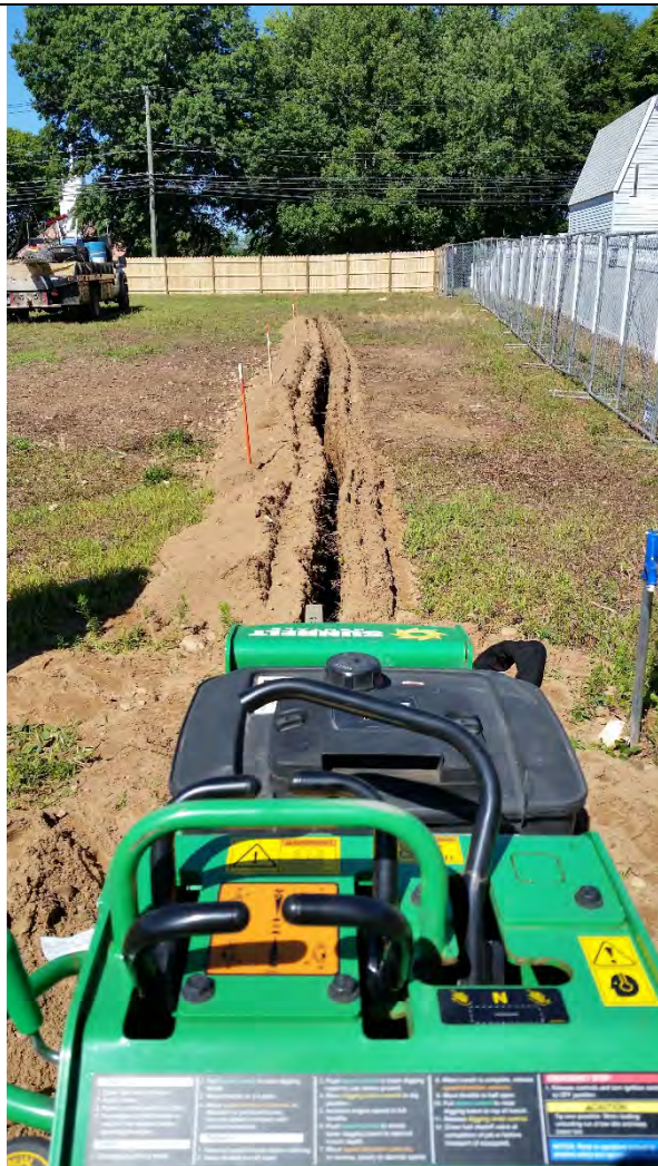
Trench for underground electric service.
