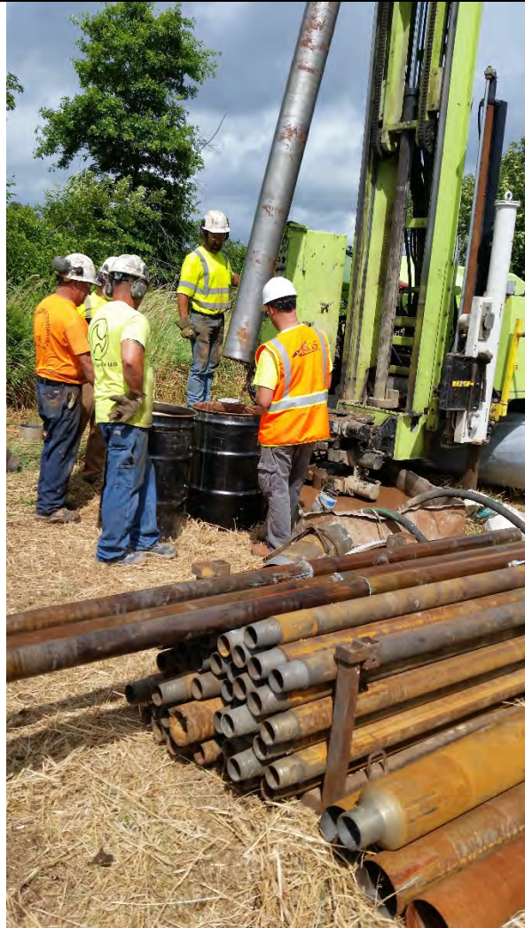
Containerizing overburden cuttings - MW-10.
