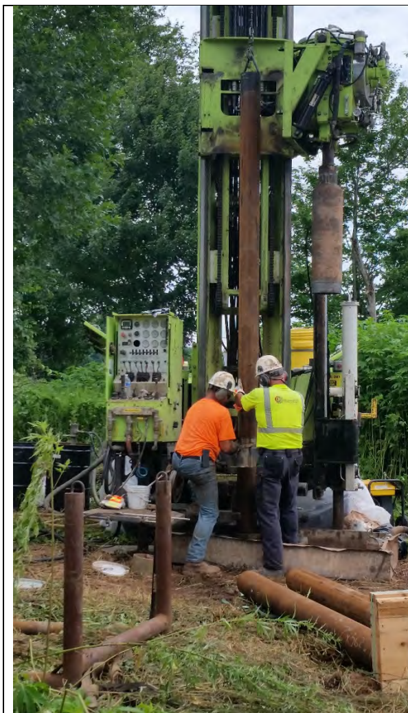
Installing permanent 6-inch casing – MW-1.
