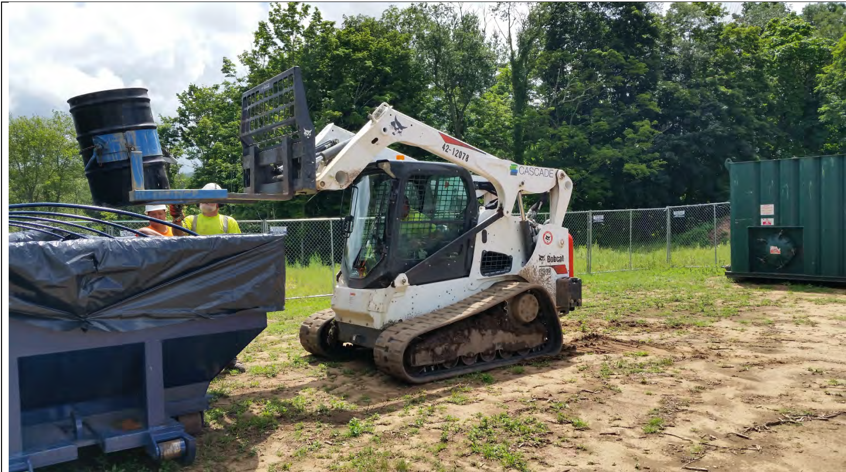
Soil drill cuttings consolidation in Staging Area roll-off container.
