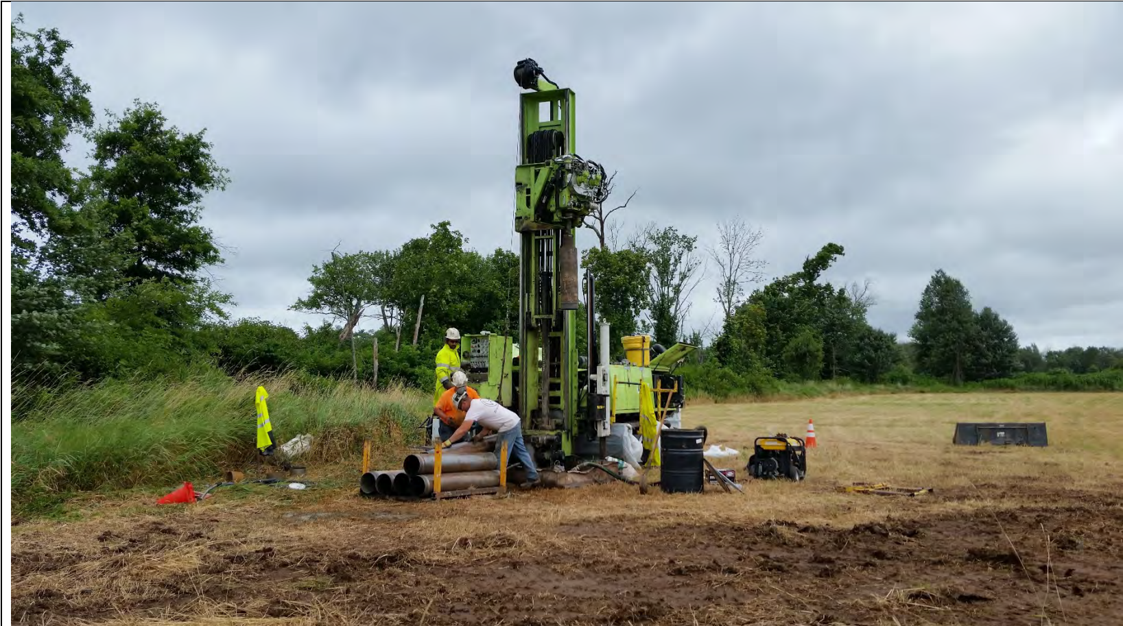
Drilling overburden with 9-inch temporary casing - MW-10.
