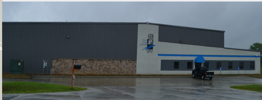
Warehousing space at the site.
