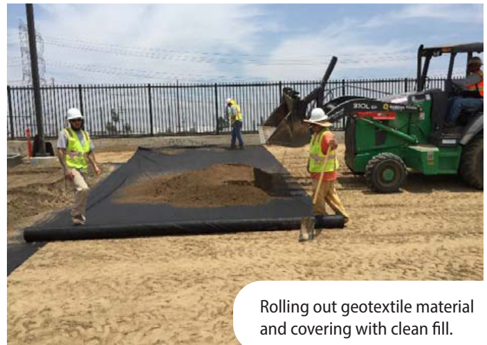
Subgrade earthwork on site.
