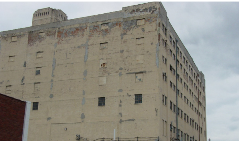
The building before demolition, cleanup and redevelopment on the site.
