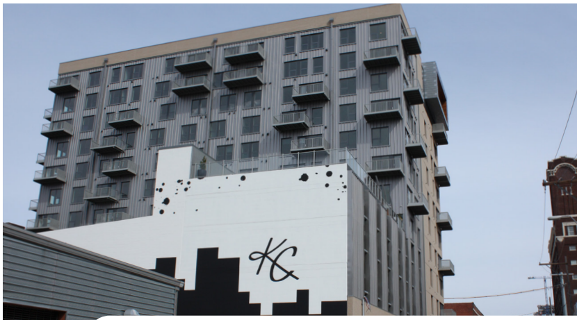
The newly constructed apartment complex after demolition, cleanup and redevelopment on the site.
