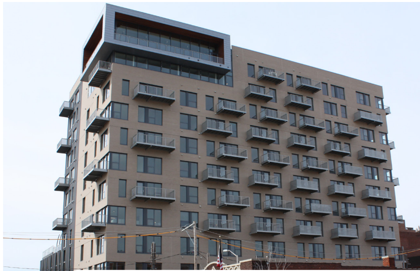
The newly constructed apartment complex after demolition, cleanup and redevelopment on the site.
