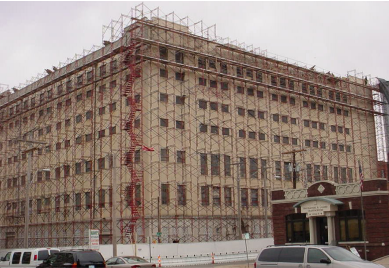
The building before demolition, cleanup and redevelopment on the site.
