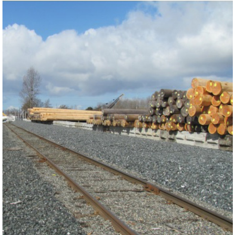
Gravel cover and railroad access at the Oeser Company's woodtreatment facility.
