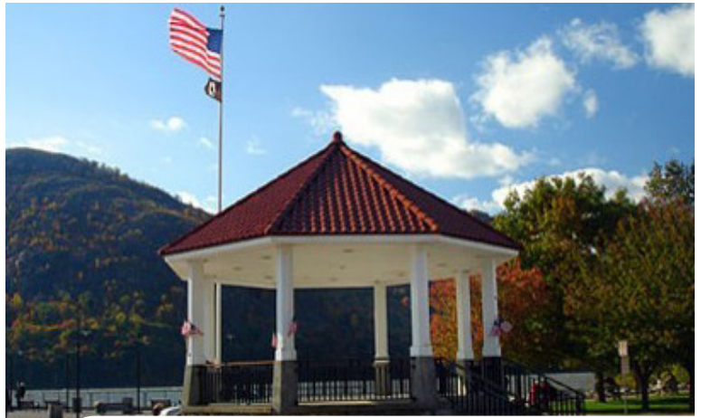
Village of Cold Spring Pier after restoration.
