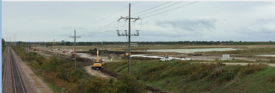
Cleanup in progress at the site.
