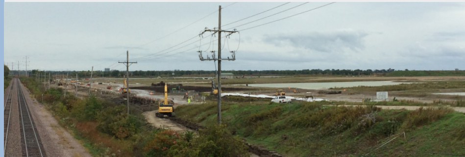
Cleanup in progress at the site.
