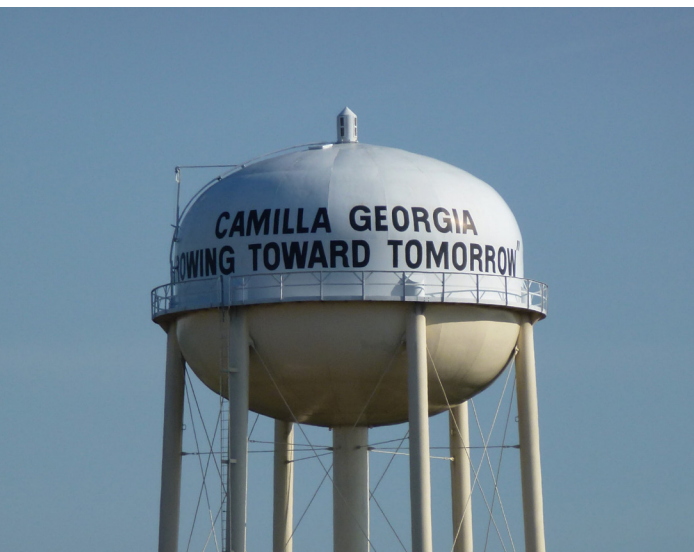
The Camilla Water Tower, visible from the recreation complex at the site.
