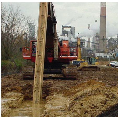
Excavation of a slurry wall trench.
