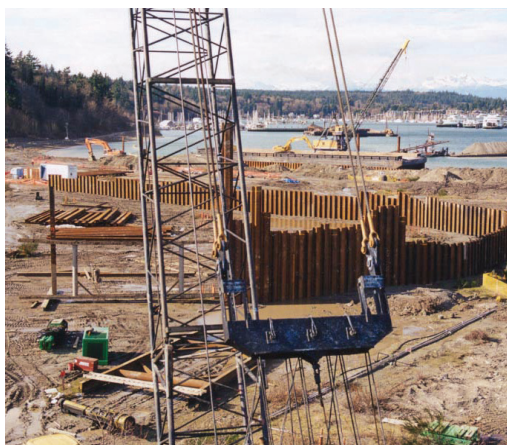
Installation of sheet piling.
