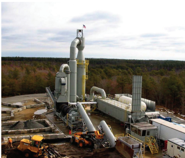
Onsite thermal desorber.
