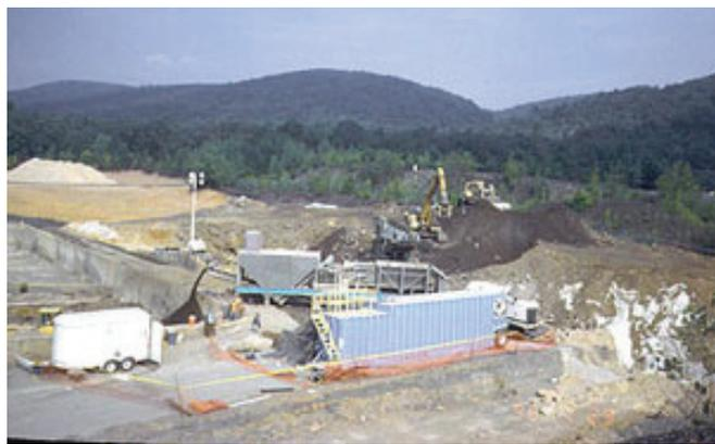
*Contaminated soil mixed with cement in a pug mill is spread on the ground as pavement.*
