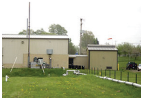
Groundwater treatment building
