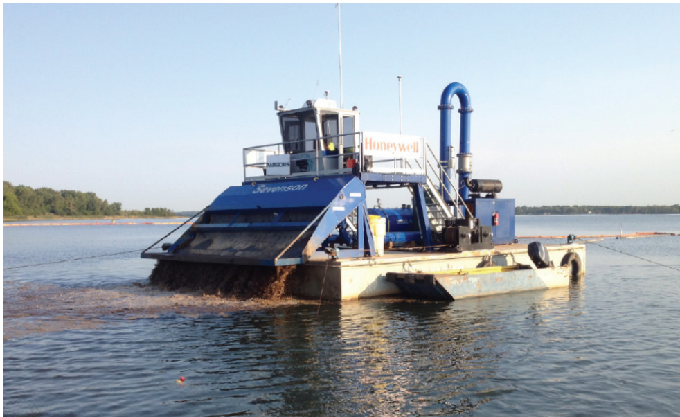
Barge pouring activated carbon onto lake sediments.
