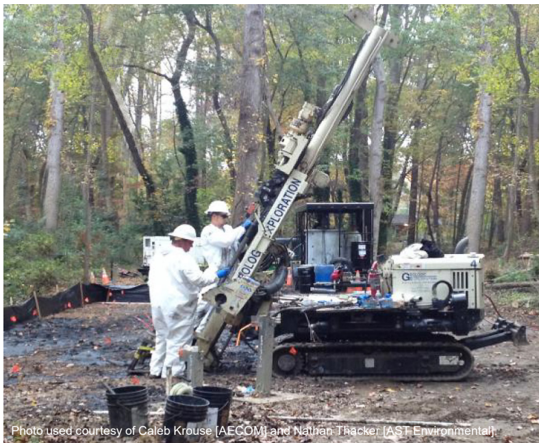
Injecting amendments at angle underground.
