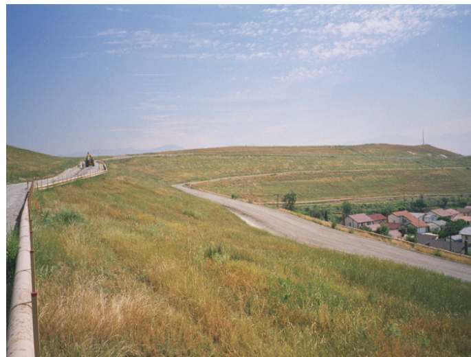
Example of ET cover used at Operating Industries, Inc. Landfill Superfund site.
