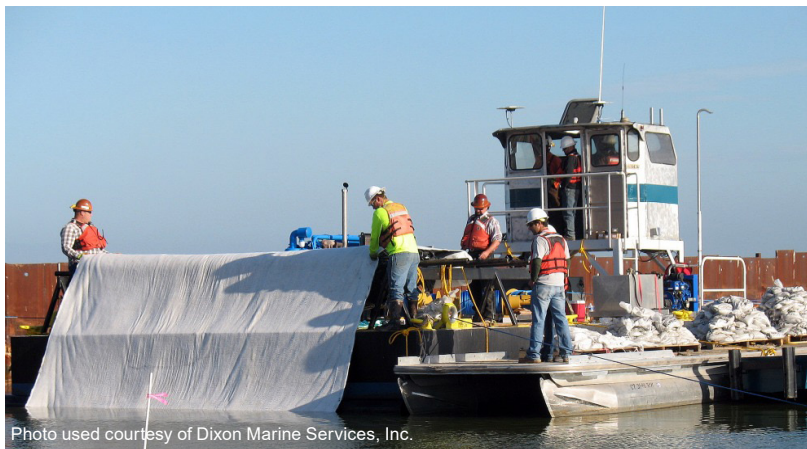
Placement of an amendment mat containing organoclay.
