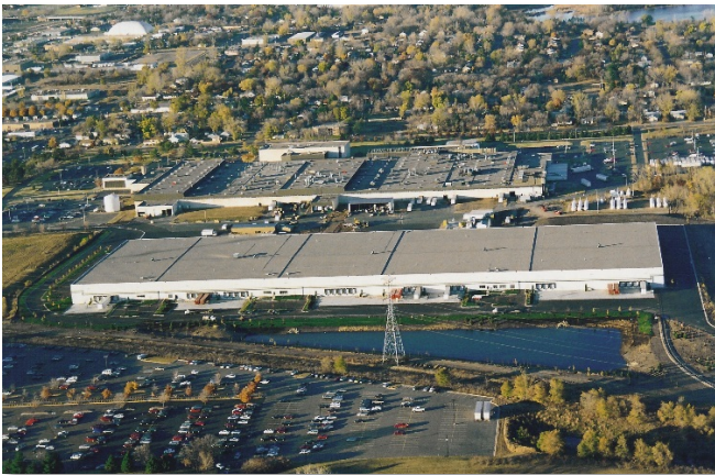
Figure 9. Aerial view of the Murphy Warehouse Company facility. Image source: Murphy Warehouse Company
