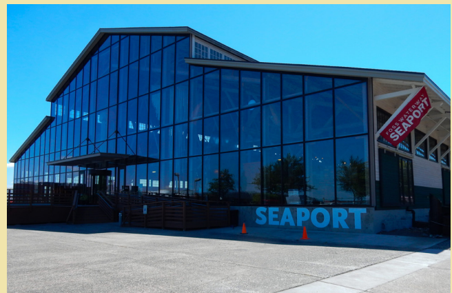
View of the restored Foss Waterway Seaport facility.
