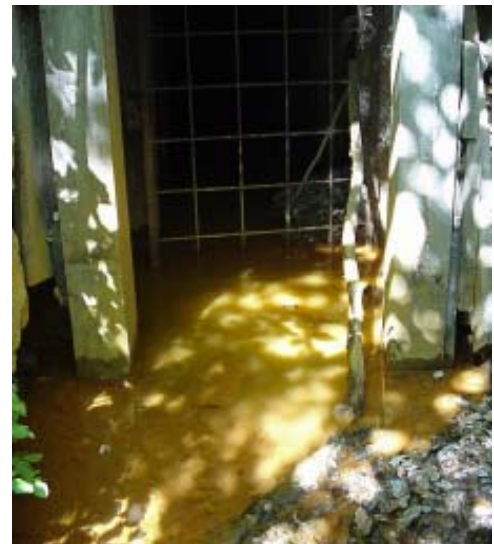
Acid mine drainage leaking from the Stowell portal at Mammoth Mine, California.
