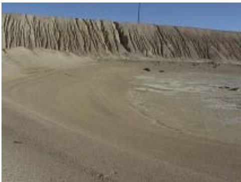
Wind and water erosion of tailings piles at Anaconda Mine, Yerington, Nevada.
