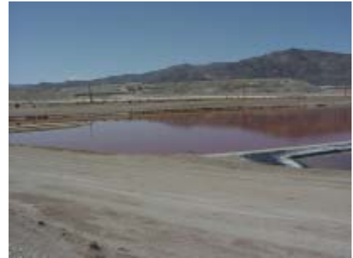
Unlined leachate and contaminated ground water evaporation ponds at Anaconda Mine, Yerington, Nevada.
