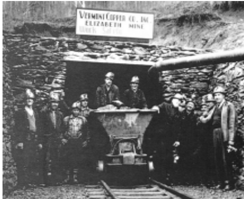
Historical mine portal at Elizabeth Mine, Strafford, Vermont.
