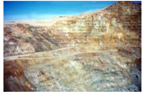
Highwall at Golden Sunlight Mines near Whitehall, Montana.
