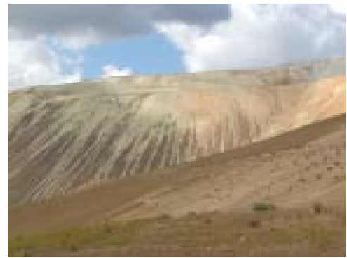
Erosion on mine tailings ponds at Kennecott Copper Mine, Magna, Utah.
