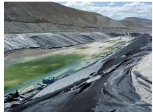
Inactive copper leachate collection pond adjacent to heap leach pile (left) at the Anaconda Mine, Yerington, Nevada.
