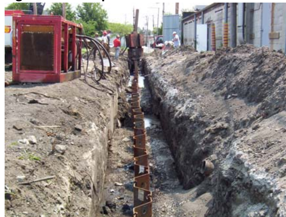
Figure 6. Sheet pile Electrode Installation
