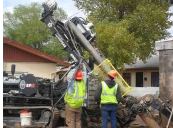
Figure 6. Sheet pile Electrode Installation
