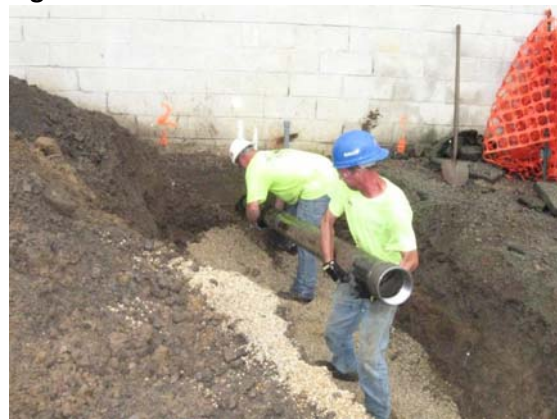
Figure 7. Horizontal Electrode Installation
