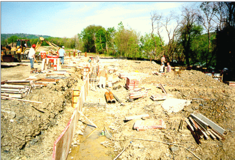
Construction of a slurry wall at the Ohio River Park Superfund site in Neville Island, Pennsylvania.
