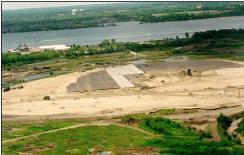
Part of the Enterprise Avenue site at the Philadelphia International Airport is covered with a concrete runway capable of landing large aircraft.
