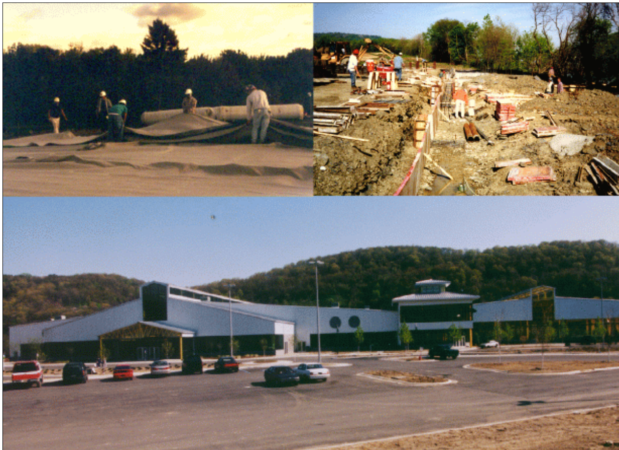
Protective cover installation, slurry wall construction, and the completed Island Sports Center.
