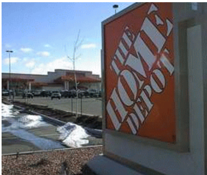
The asphalt parking lot at the Home Depot site in Denver, Colorado also serves as a protective cover for insoluble metals-contaminated soils. The contaminated soils were consolidated into four containment cells.
