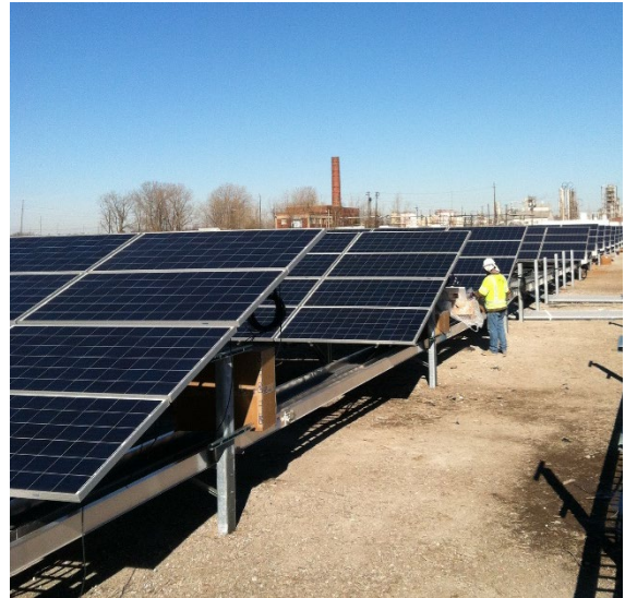
Figure 9. Driven-pile Anchoring System at the Reilly Tar Superfund Site, Indianapolis, Indiana. Source: EPA.
