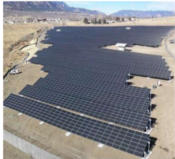
Figure 7. Ballasted solar system. Source: NREL.
