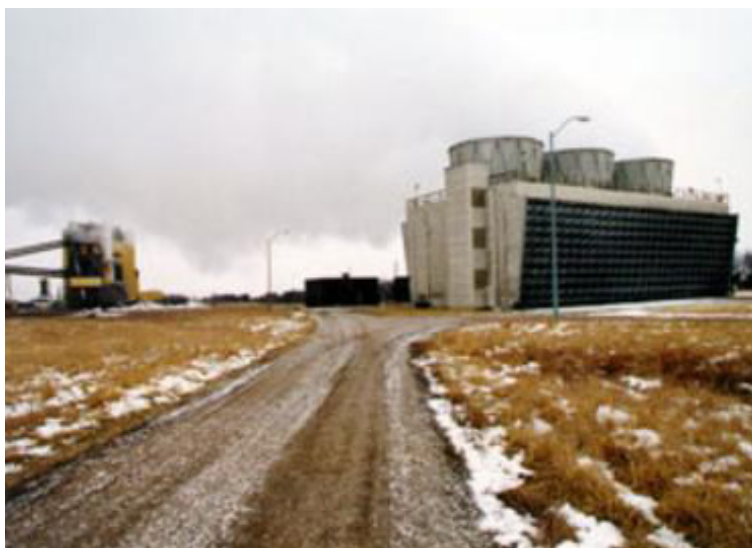
Figure 17. Extracted groundwater is used as cooling water at the coal-fired power plant at the Whelan Energy Center at the Hastings Ground Water Contamination Superfund site (Nebraska).
