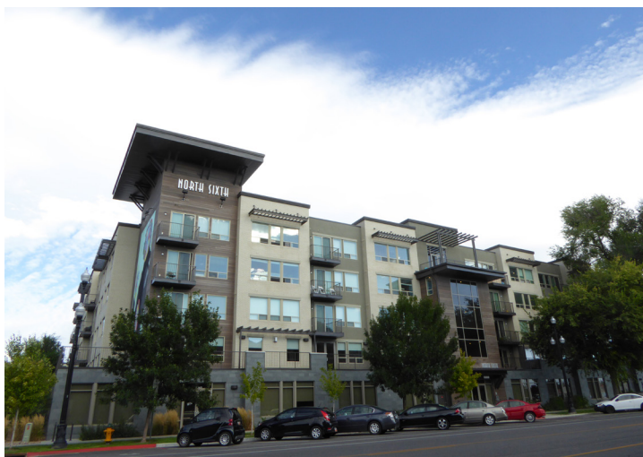
Figure 2. The North Sixth commercial building at the Utah Power & Light/American Barrel Co. Superfund site (Utah, Region 8).
