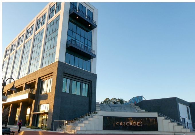
Figure 10. A commercial building at Cascades Park at the Cascades Park Gasification Plant site (Florida, Region 4).
