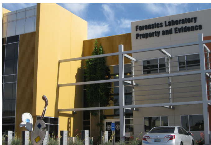
Figure 21. The Scottsdale Police Department Forensics Lab at the Indian Bend Wash Area Superfund site (Arizona, Region 9).
