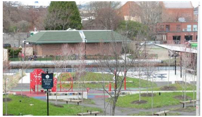
Figure 115. The Peabody Street Park/Harborwalk at the Peabody Street Asbestos site (Massachusetts).
