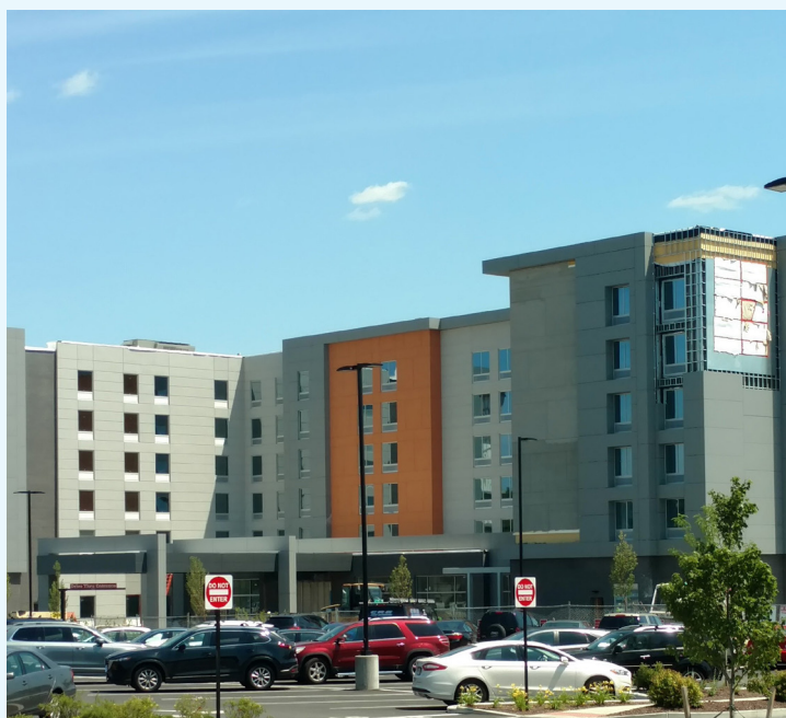
Figure 2. A new hotel at the W.R. Grace property at the Wells G&H site (Massachusetts).
