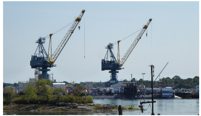
Figure 72. Naval facilities at the Portsmouth Naval Shipyard site (Maine).
