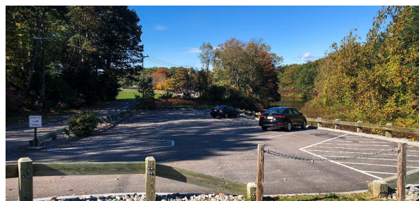
Figure 16. The parking lot at the Fletcher's Paint Works & Storage Superfund site, built to improve public access to Keyes Memorial Park (New Hampshire).
