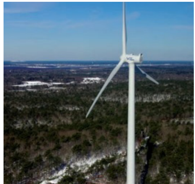
Figure 106. One of three 1.5-megawatt turbines used to offset electrical costs for powering multiple groundwater cleanup systems at the JBCC site (Massachusetts).
