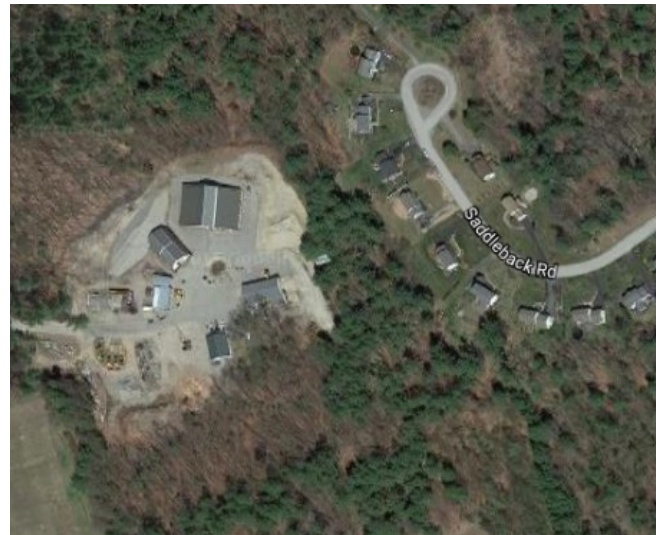
Figure 127. Aerial view of the Town Garage/Radio Beacon site (Massachusetts). Sources: Imagery ©2022 Google, Imagery ©2022 MassGIS, Commonwealth of Massachusetts EOE, Maxar Technologies, USDA/FPAC/GEO, Map data ©2022.
