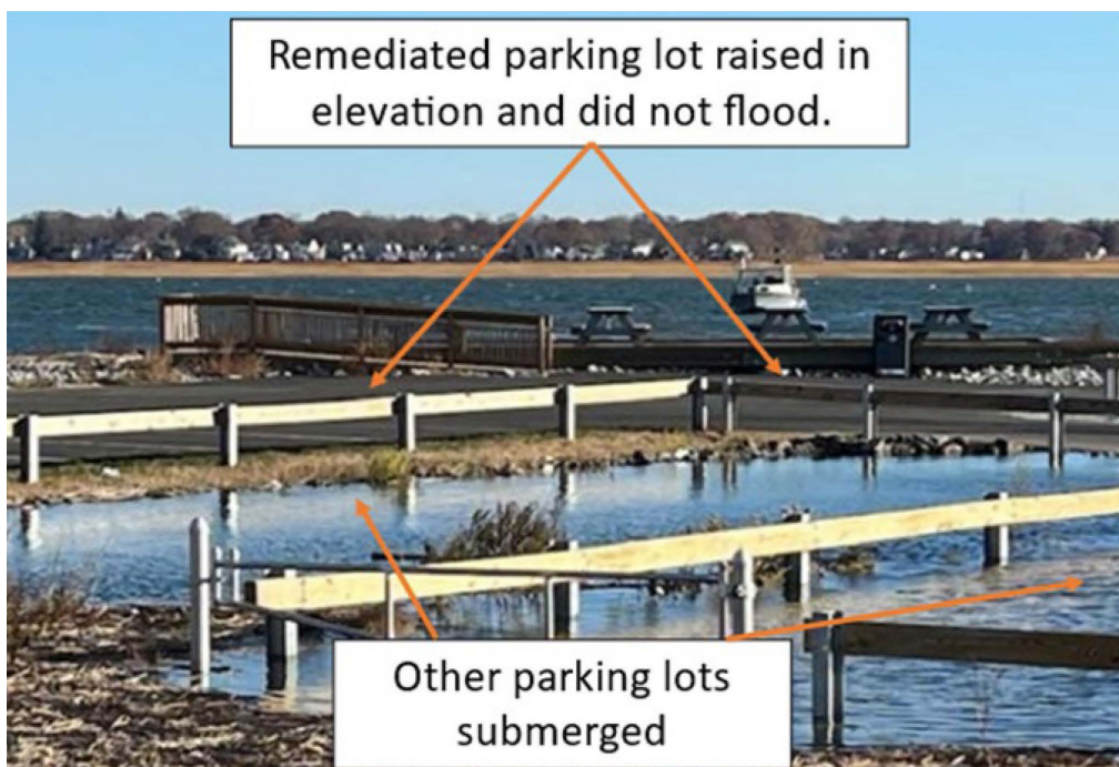
Figure 33. EPA cleanup raised a portion of docks and parking lots and improved climate resiliency at the restored Beacon Point (Connecticut).
