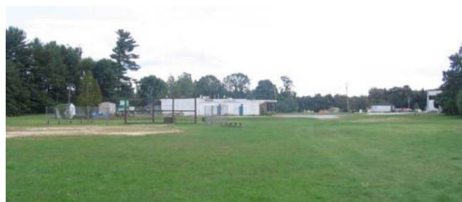
Figure 123. Recreational facilities include a baseball diamond and open space at the Savage Municipal Water Supply site (New Hampshire).
