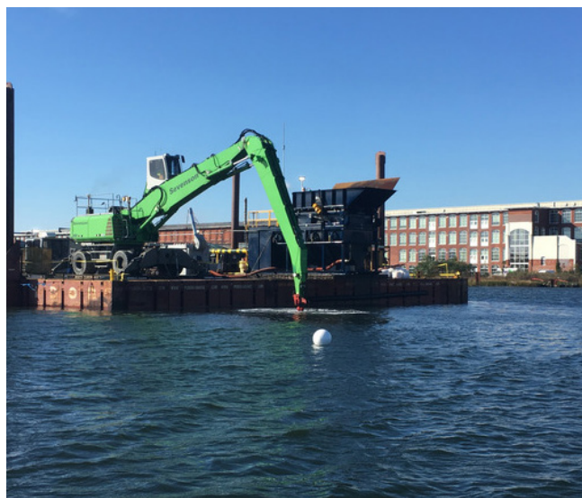
Figure 87. Dredging of contaminated sediment has helped pave the way for commercial port development at the New Bedford Harbor site (Massachusetts).
