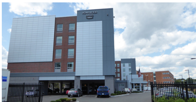
Figure 44. Lawrence Metals site (Massachusetts).
