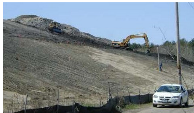
Figure 82. Soil grading and shaping of the landfill at the Haverhill Municipal Landfill site (Massachusetts).
