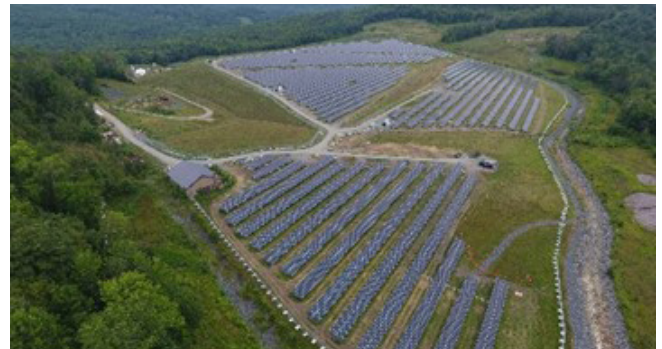
Figure 142. Solar array at the Elizabeth Mine site (Vermont). Image used with permission of Weston and Sampson, Conti Solar, and Elizabeth Mine Solar.
