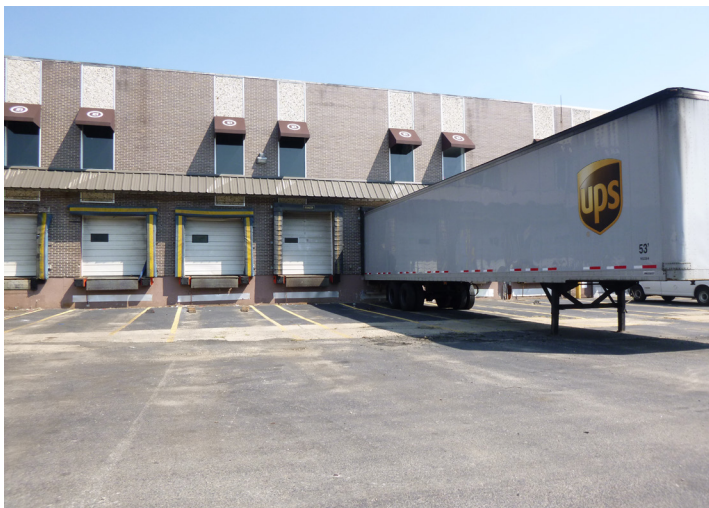
Figure 7. A distribution warehouse at the Peterson/Puritan, Inc. site (Rhode Island).
