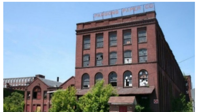
Figure 114. View of the Parsons Paper Mill site (Massachusetts) prior to demolition.
