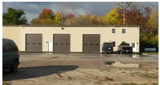
Figure 120. The Kearsarge Metallurgical Corp. site's former groundwater treatment building is now home to an automobile workshop (New Hampshire).
