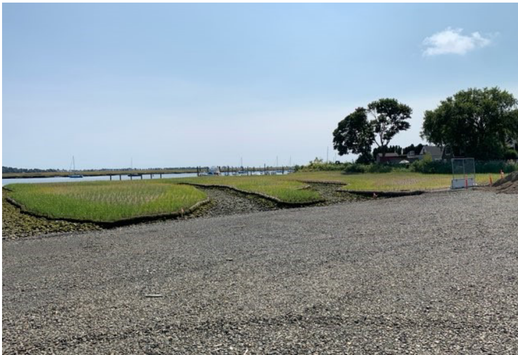
Figure 32. Lockwood Avenue Wetland after cleanup and restoration (Connecticut).
