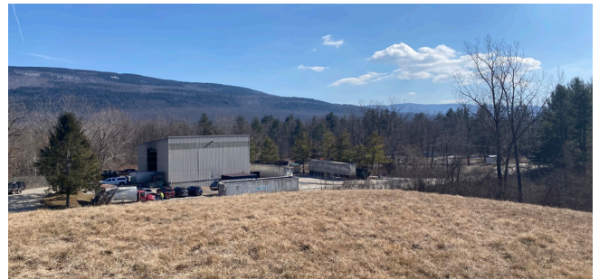
Figure 140. A waste and recycling service station at the Bennington Municipal Sanitary Landfill site (Vermont).
