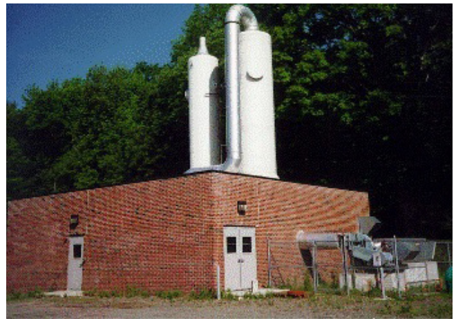
Figure 125. The groundwater treatment facility at the South Municipal Water Supply Well site (New Hampshire).
