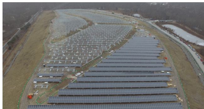
Figure 135. Aerial view of solar facility at the Rose Hill Regional Landfill site (Rhode Island). Photo used with permission of Kearsarge Energy.
