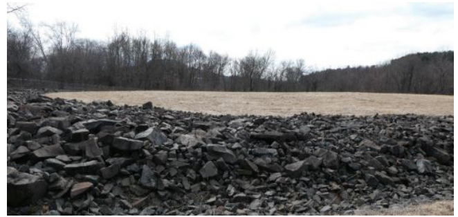
Figure 91. Drainage along the capped area of the PSC Resources site (Massachusetts).
