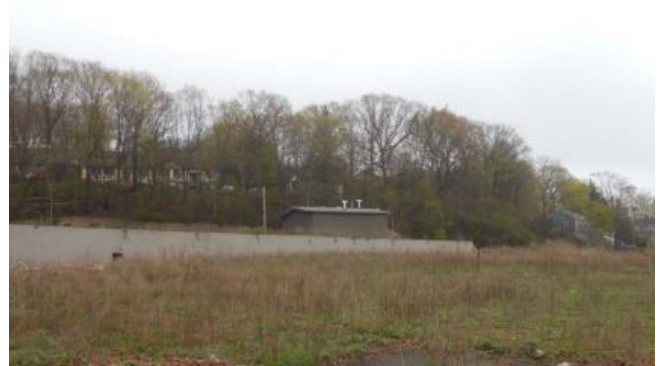
Figure 52. The groundwater treatment building at the Kellogg-Deering Well Field site (Connecticut).
