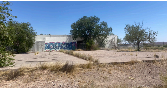
Figure 7. Manufacturing Building (Zone A).
