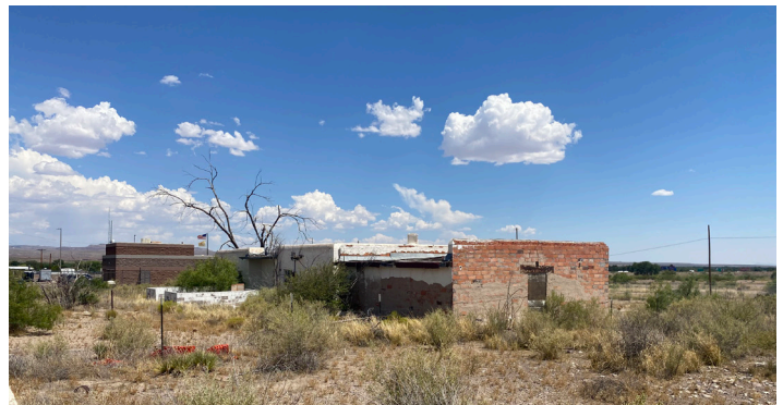
Figure 8. Area west of NM State Police Station (Zone A2).
