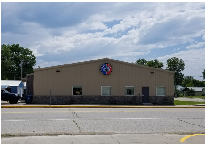
Figure 4: Environmental Realty Building.
