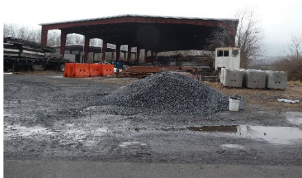
A storage shed at the Drake Site.
