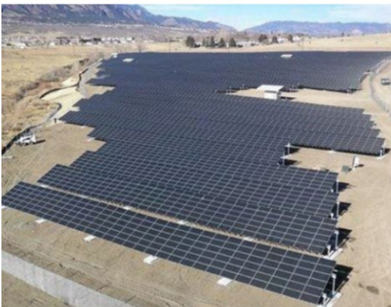
Fig. 7 Ballasted solar system. Source: NREL.
