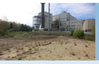
The largest alternative energy facility is Greenleaf Power's Plainfield Renewable Energy biomass cogeneration plant at the Gallup's Quarry Superfund site in Plainfield, Connecticut. The 37.5-megawatt facility uses waste wood to generate enough electricity to power the equivalent of about 40,000 homes in Plainfield. The facility provides a market for waste biomass materials that would otherwise be taken to a landfill or left to decay, leading to off-gassing of methane and other greenhouse gases.
