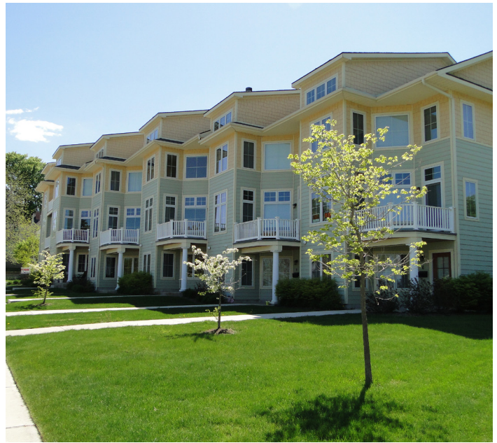
Figure 9. Condominium complex and recreational trail at the PMC Groundwater site (Michigan, Region 5).
