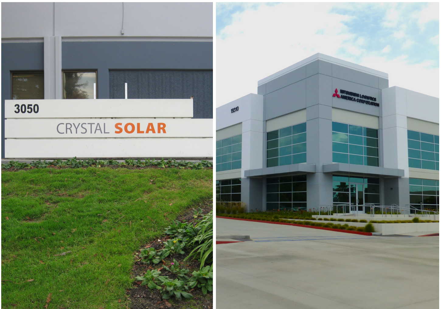
Figure 3. Business offices at the Synertek, Inc. (left) and Del Amo (right) sites (California).
