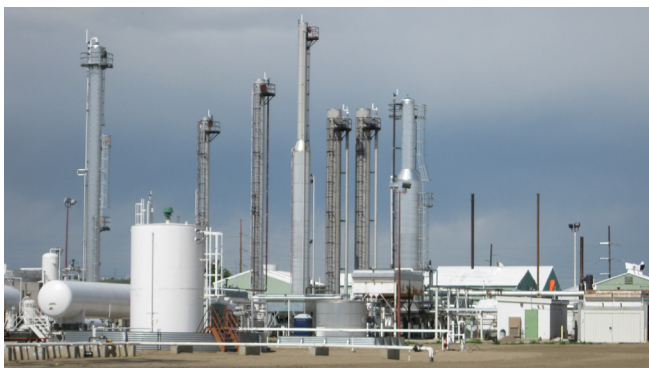
Figure 28. Mystery Bridge Road/U.S. Highway 20 (Wyoming).
