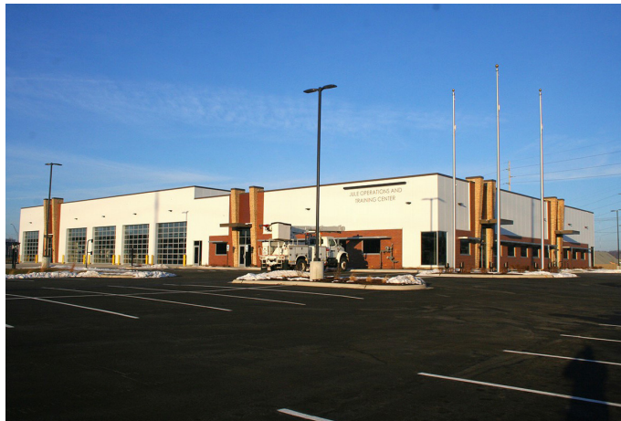
Figure 8. An operations and training center at Peoples Natural Gas Co. site. (Iowa).
