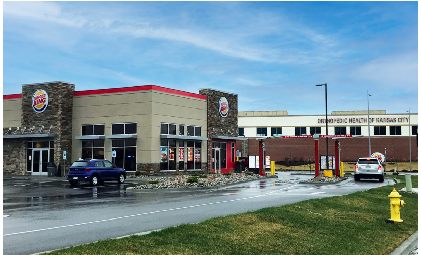
Figure 22. A fast food restaurant at the Armour Road site (Missouri).
