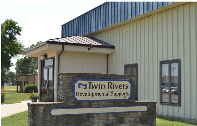
Figure 7. An agency for individuals with developmental disabilities at the Strother Field Industrial Park site (Kansas).
