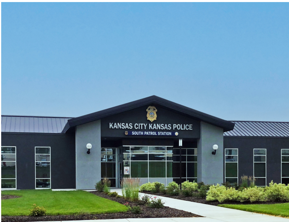
Figure 16. The design of the South Patrol police station encourages community interactions at the Kansas City Structural Steel site. (Kansas)
