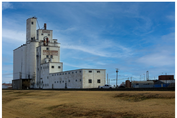
Figure 2. A local utility maintenance yard sits at the foot of an old grain silo at the City of Perryton Well No. 2 site (Texas).
