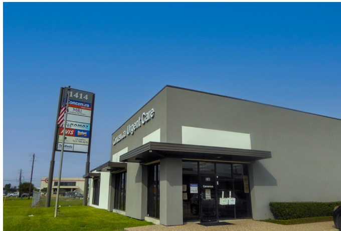
Figure 8. Store front and sign at the Sol Lynn site (Texas).
