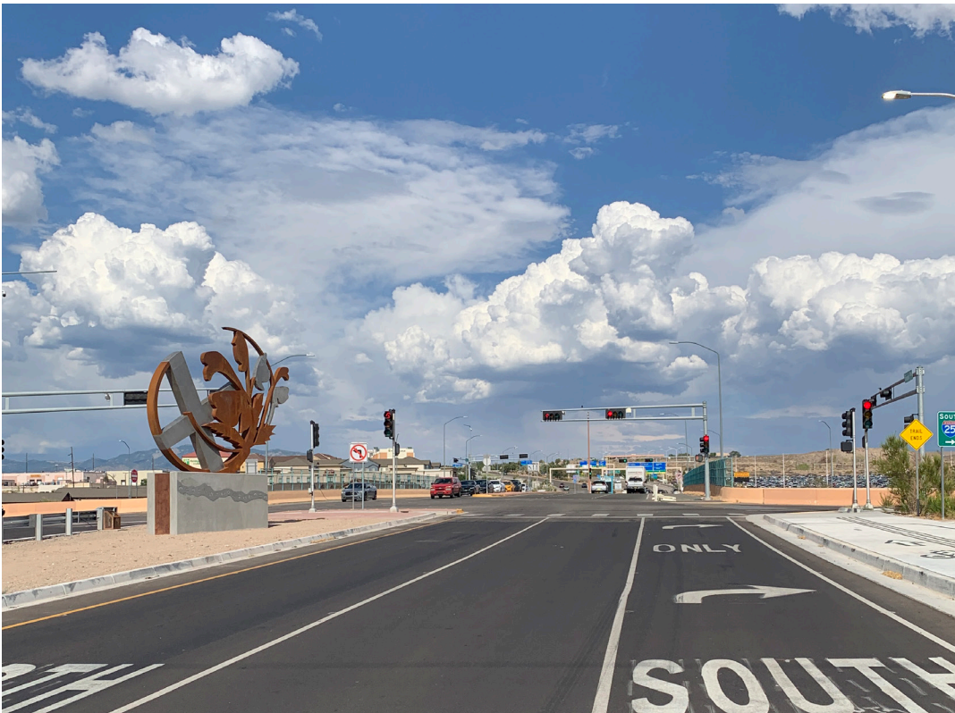
Figure 19. The new Sunport Boulevard extension closes a gap in the area’s transportation network, and address other transportation and access needs on and around the South Valley Superfund site (New Mexico).
